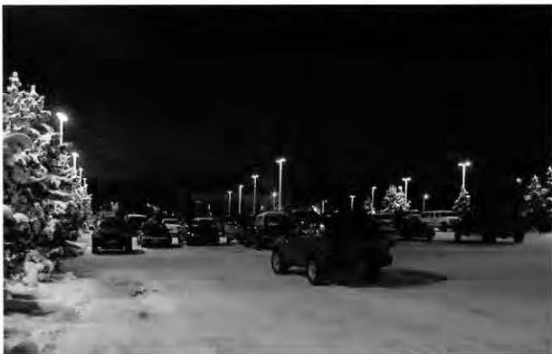
Figure 12: Parking Lot in LZ 2 - Fully shielded, uniform distribution. Anchorage, AK (Image courtesy of N. Clanton)
