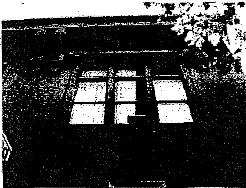
Detail of window and cornice
