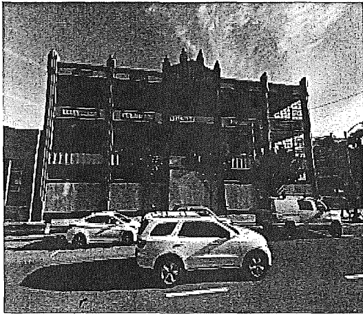
Eng-Skell Building (1035 Howard Street, 1930)
