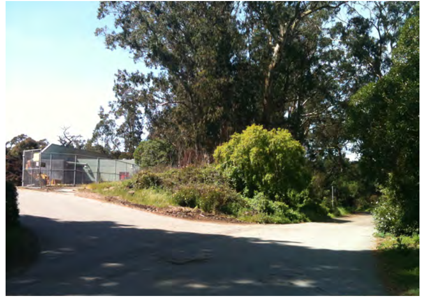
Photo 12 - West-facing View along Overlook Drive toward Central Pump Station
