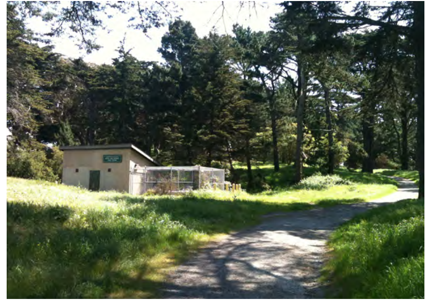
Photo 18 - East-facing View of the Existing North Lake Well Facility Site from Park Access Road
