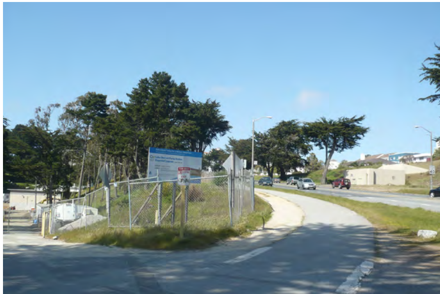
Photo 3 - North-facing View of Site Access Road and Lake Merced Boulevard from Lake Merced Boulevard Sidewalk
