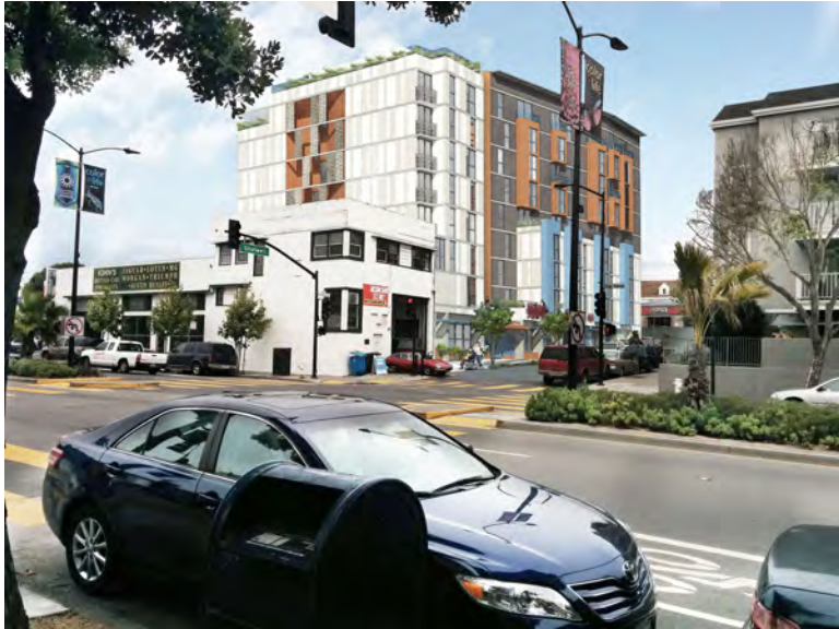
View from SE Corner
