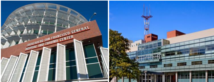
ZSFG & LHH Critical Repairs & Renovations
