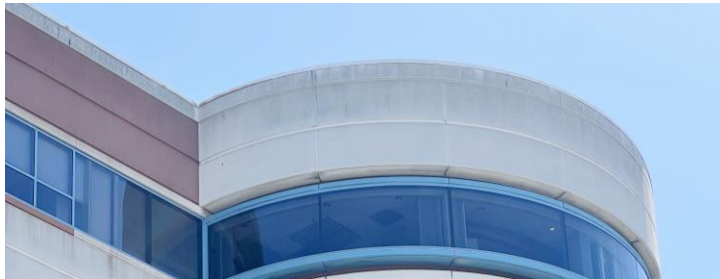
ZSFG Building 3 Retrofit
