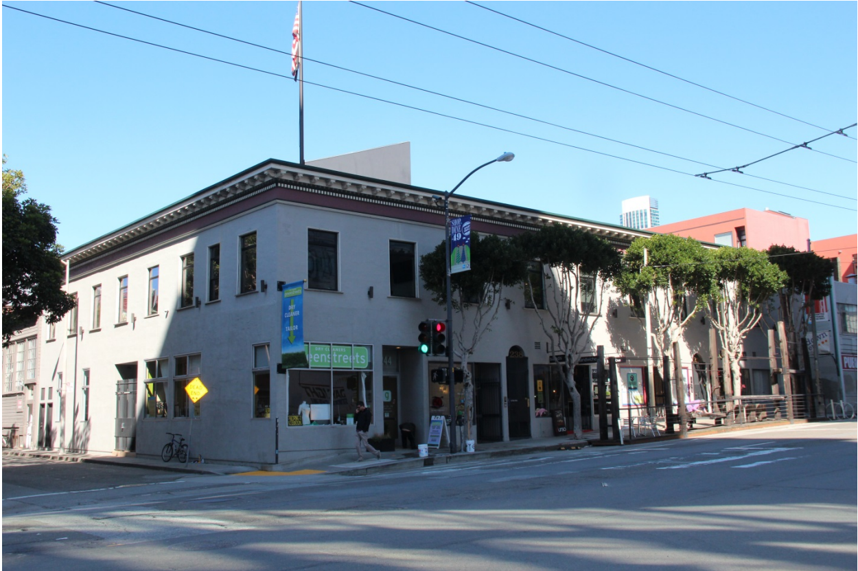
228-248 TOWNSEND STREET NEW PULLMAN HOTEL
