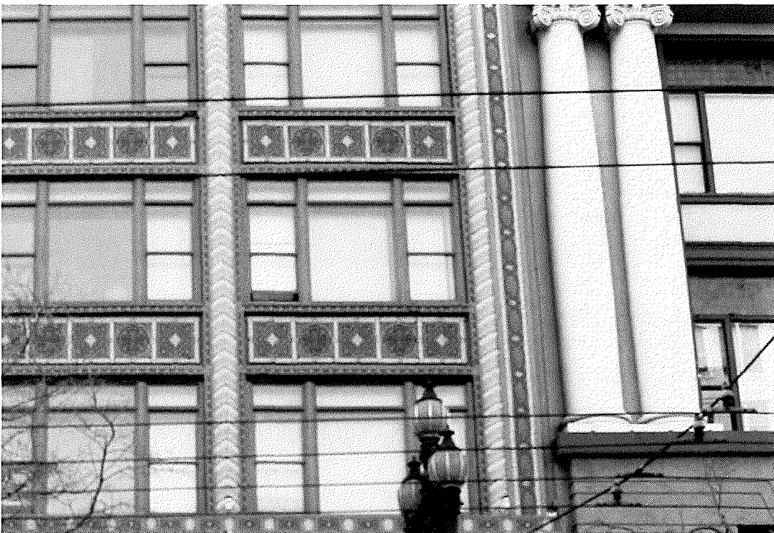
10. April 2017, Exterior Detail, North Elevation, Third Floor, Window at West, Looking S
