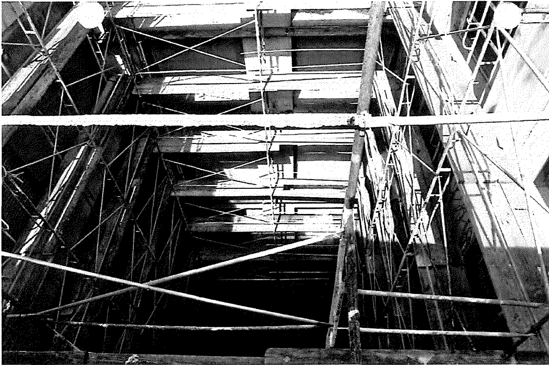
31. April 2012, Lightwell at Center-West, Looking W
