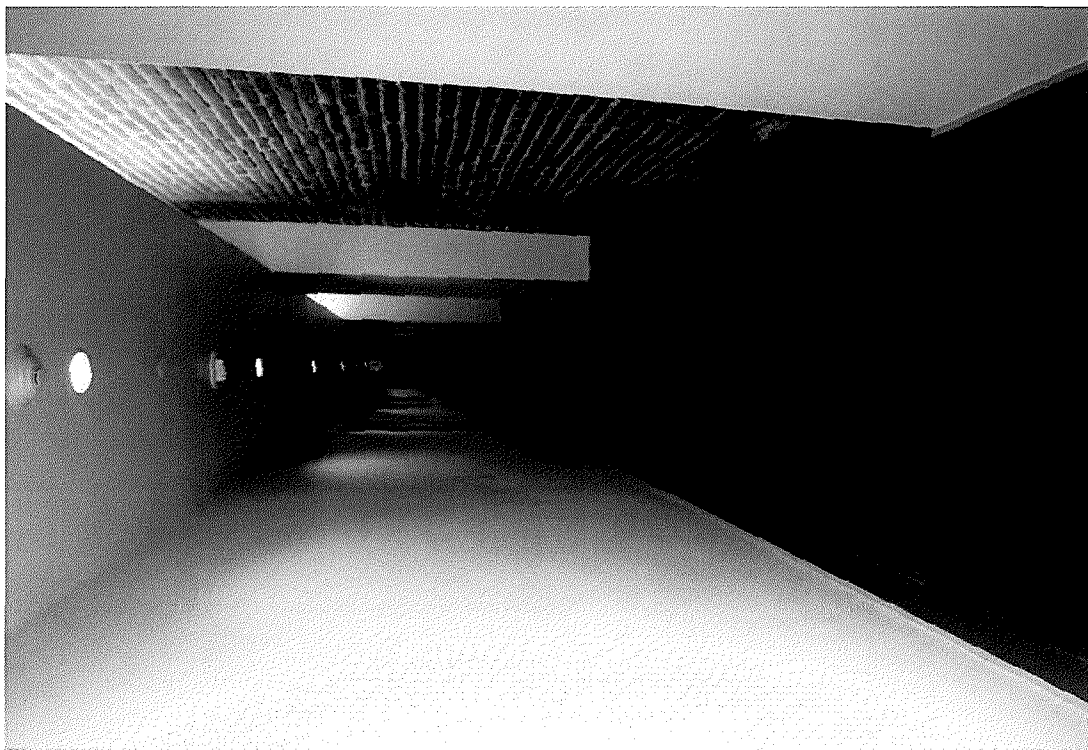
38. April 2017, Additional Photographs, Typical Corridor at East, Looking N
