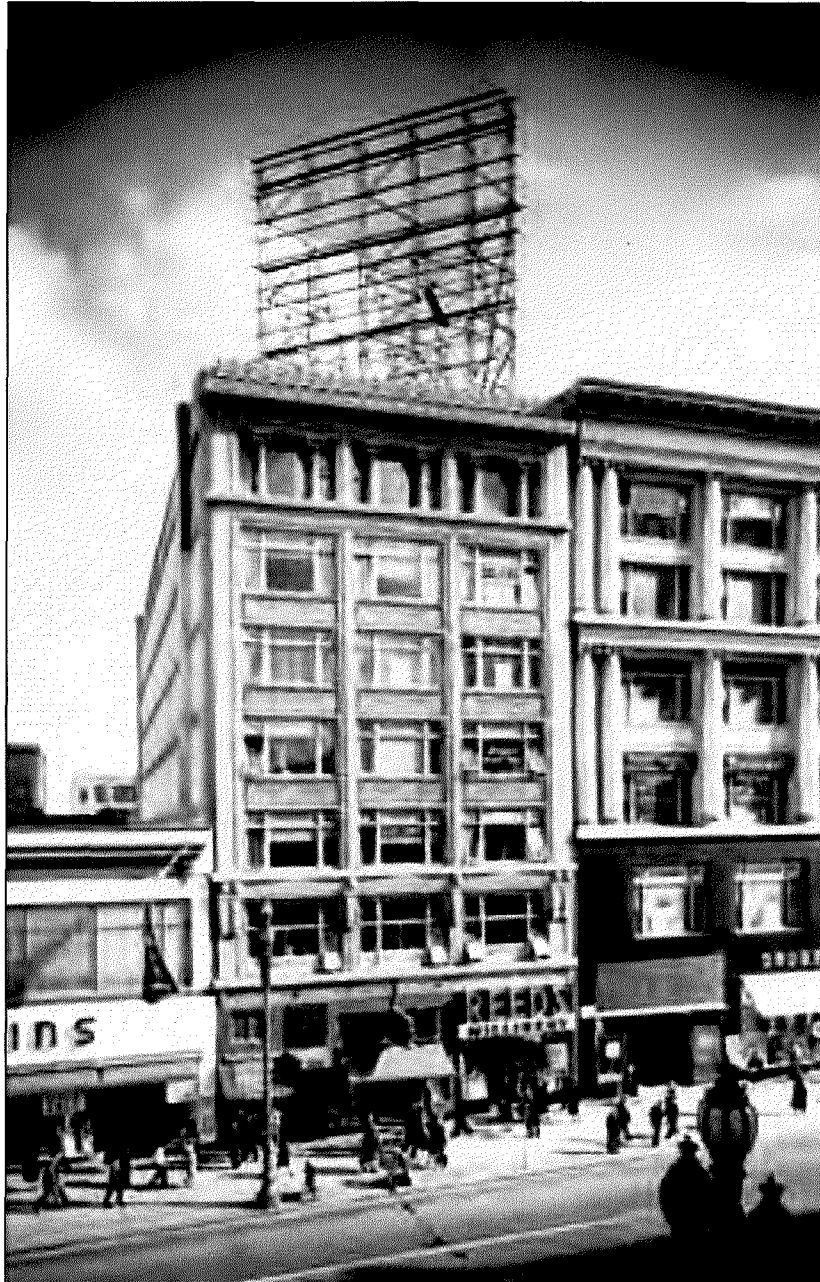
Wilson Building, May, 1944
