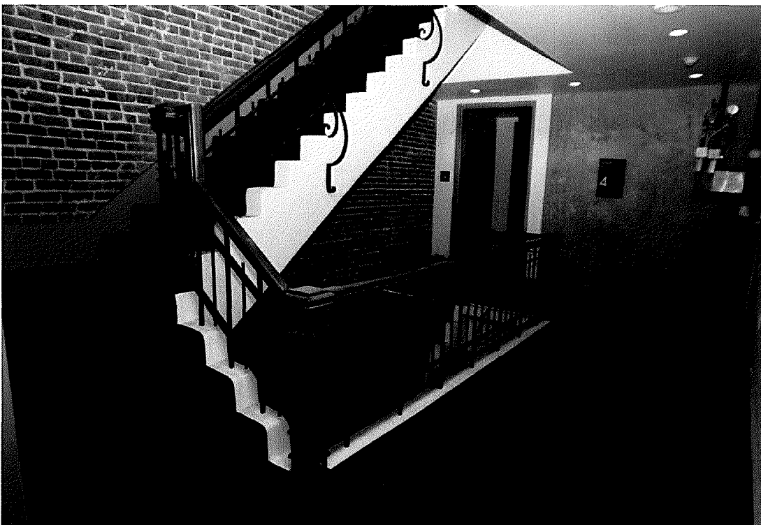
28. April 2017, Interior View, Fourth Floor, Stair at Center-East, Looking SE, Typical
