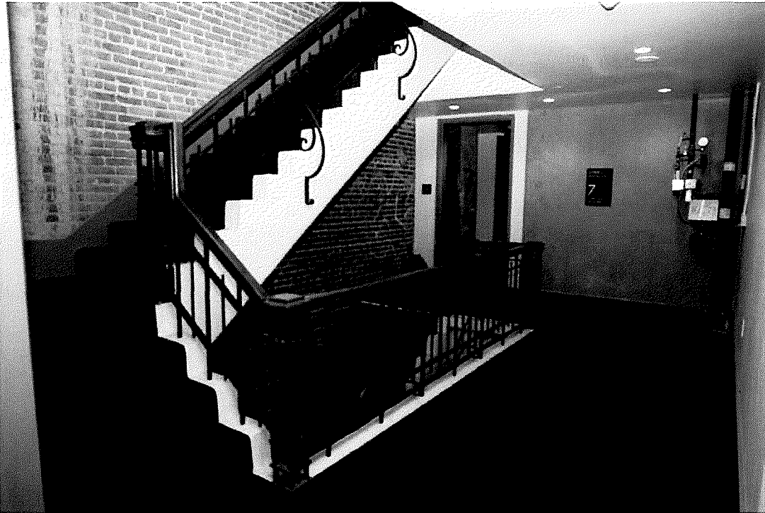
37. April 2017, Additional Photographs, Stair Landing
