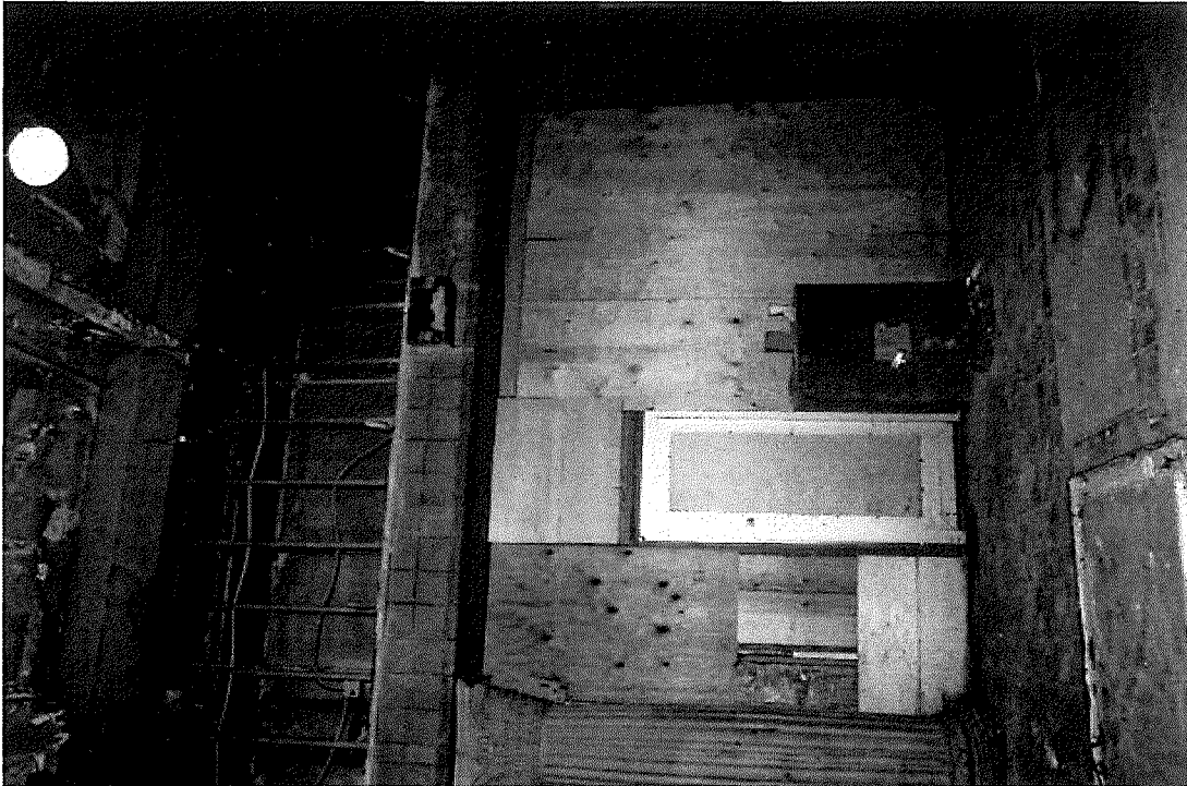
19. April 2012, Interior View, Ground Floor at Northeast, Looking N
