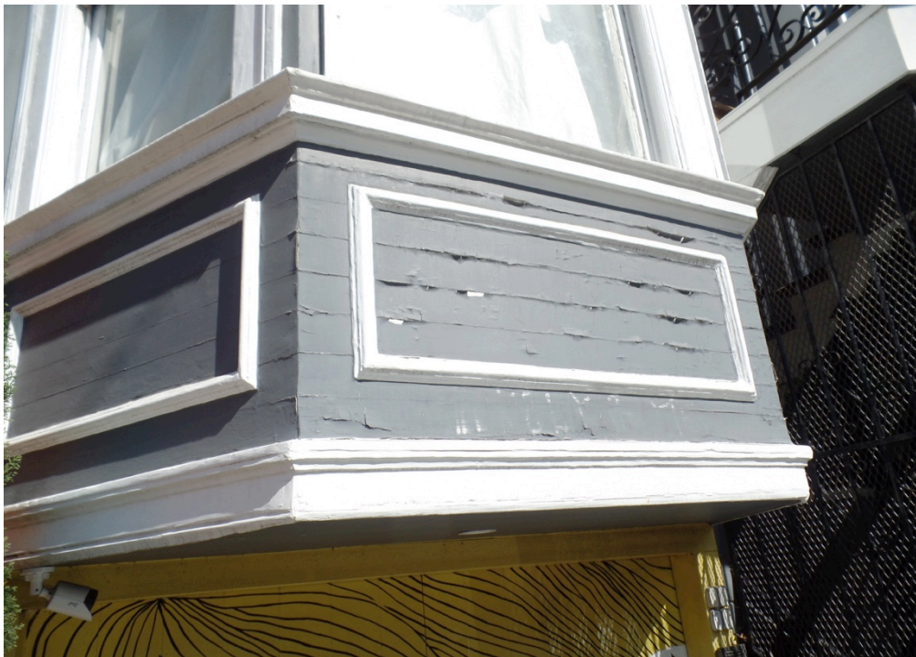
Figure 12: Front elevation view of peeling paint on bay window at second level (Garavaglia Architecture, 2022).
