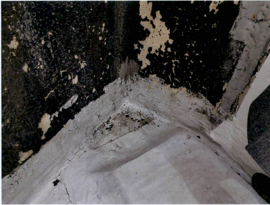
Photo 32: Failure at vertical parapet membrane – Roof.
