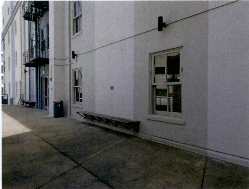
Photo N: View of north façade looking south at cement plaster coated concrete walls.
