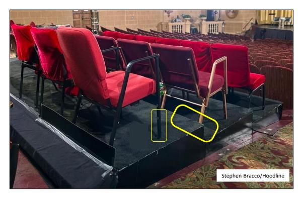
The plans replace 24 rows of 802 permanent seats with 20 rows of ~517 stackable chairs, most sitting on risers with open unprotected front edges, creating trip and fall hazards. People might step off the narrow open edges, especially in the dark. The chairs' protruding front legs create other tripping hazards. Can stackable chairs be secured safely enough for people who struggle with sitting and rising?
