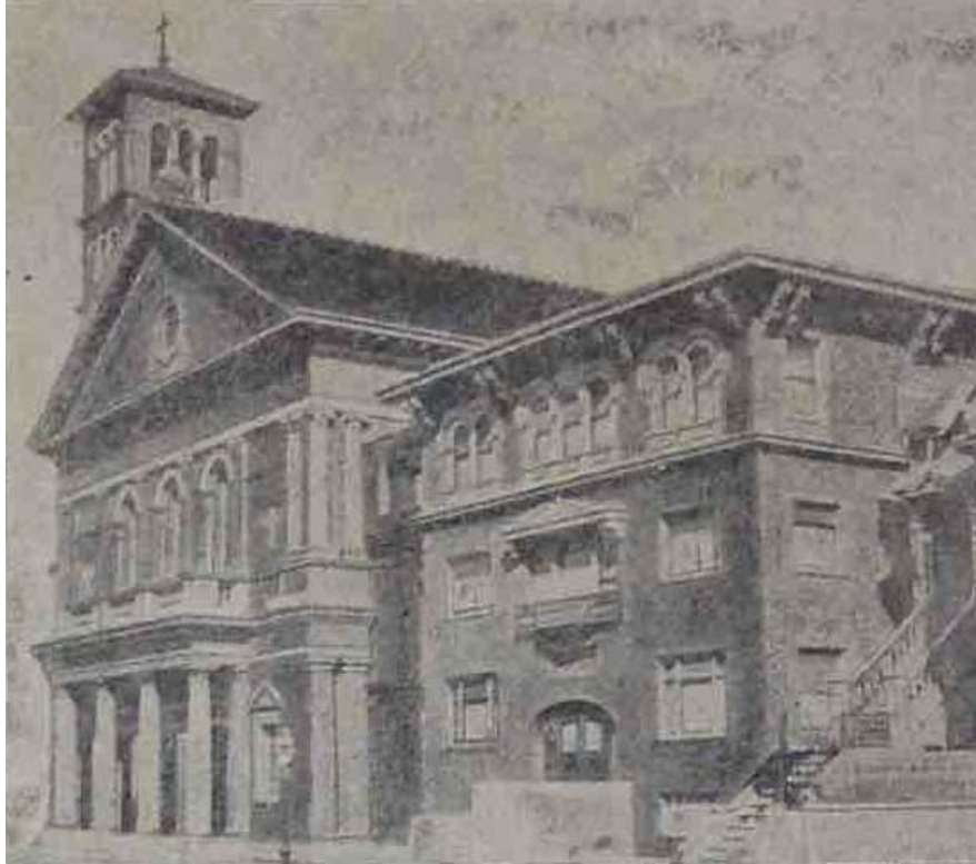
FIGURE 58. CHURCH AND RECTORY SHOWING ORIGINAL DOOR AND WINDOW TREATMENT ON FIRST AND SECOND STORIES. SOURCE: CATHOLIC MONITOR, OCTOBER 2, 1920
