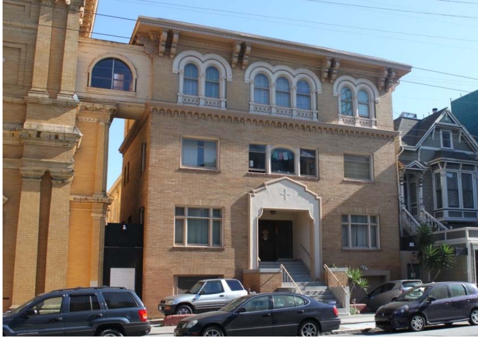
FIGURE 38. RECTORY: MAIN (WEST) ELEVATION FROM FILLMORE STREET, 2015.
