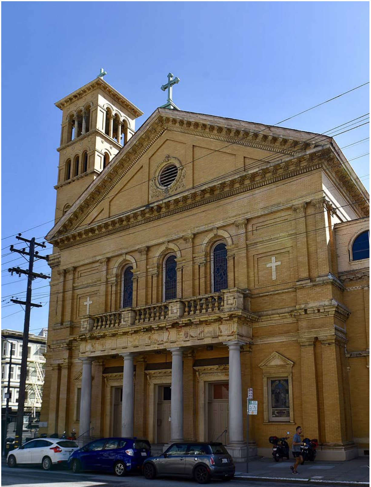
Committee February 26, 2024 Meeting Agenda 2. 231045 [Planning Code - Landmark Designation - Sacred Heart Parish Complex] Ordinance amending the Planning Code to designate the Sacred Heart Parish Complex, located at 546-548 Fillmore Street, 554 Fillmore Street, 735 Fell Street, and 660 Oak Street, Assessor's Parcel Block No. 0828, Lot Nos. 12,
