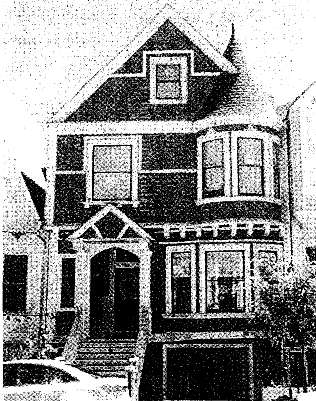
64 Pierce Street facade
