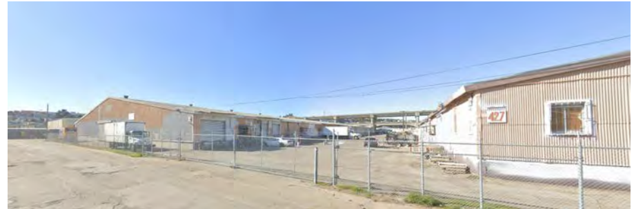
Existing View of Project Site along Rankin Street
