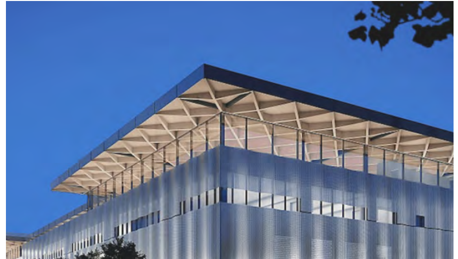
Illustrative Photo of Building with Vehicle Accessible Roof
