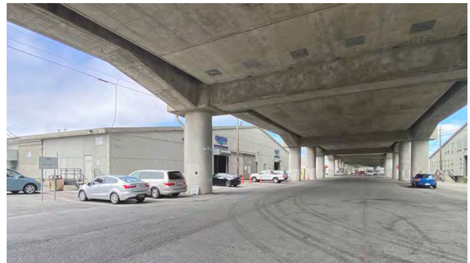
Existing View of Project Site along Selby Street
