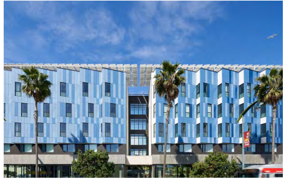
Illustrative Photo of Field Patterning with Building Materials
