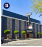
11 Bimbo's 365 Club 1001-1025 Columbus Avenue Year Built: 1981 Significant for its association with Italian American cultural heritage, its Midcentury Modern architecture designed by architect of merit Timothy Pflueger, and as a popular nightclub
