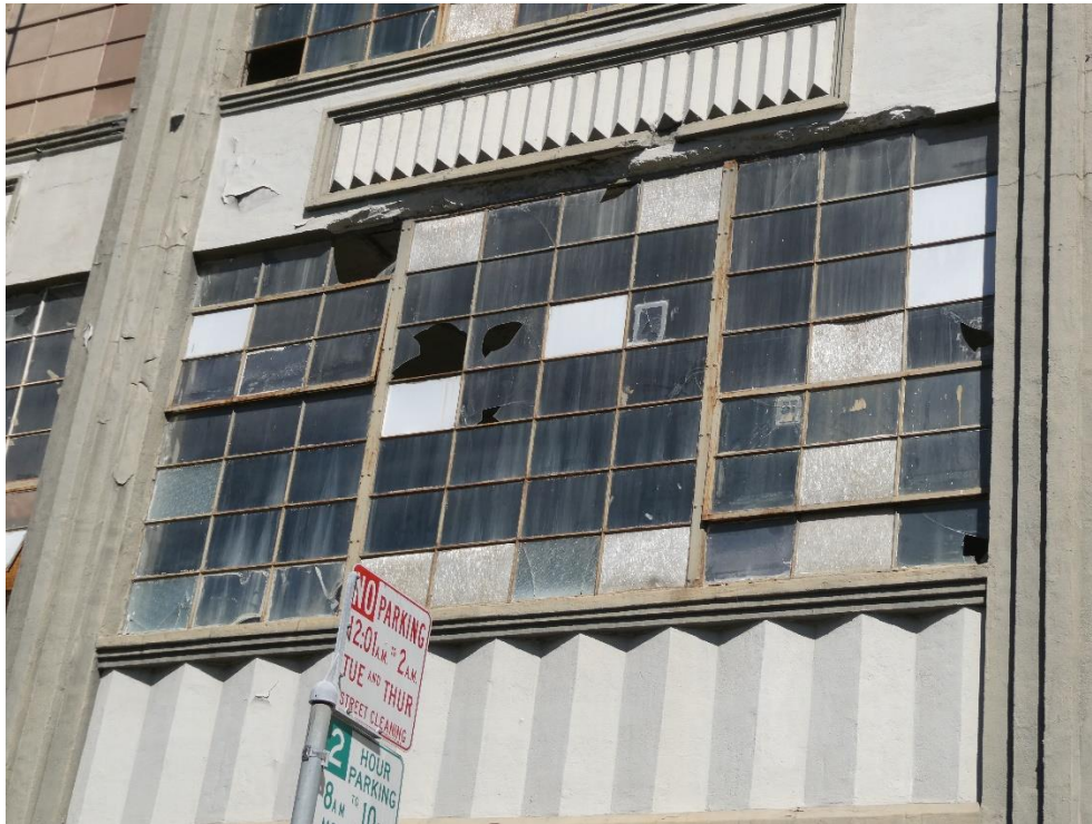
Figure 7: Additional broken and cracked panes at west façade. (Page & Turnbull, 2024)
