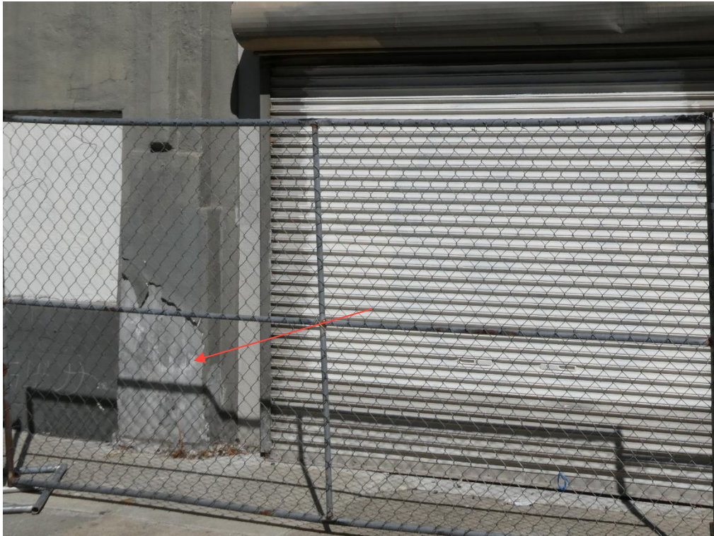
Figure 5: The stucco at this column base has delaminated and detached. (Page & Turnbull, 2024)
