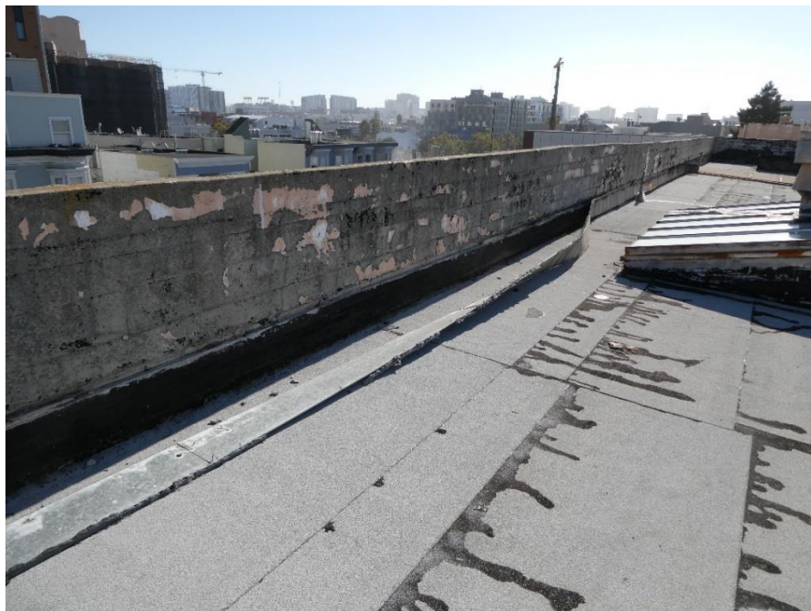
Figure 18: This area of flashing has now detached from the parapet. (Page & Turnbull, 2024)
