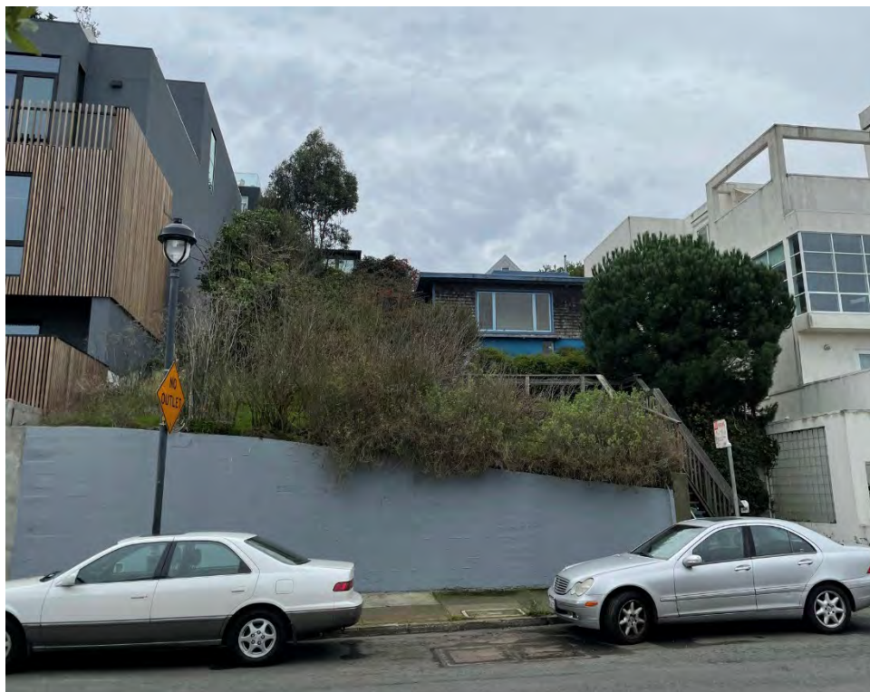
649-651 Duncan Street, view south, 2020 Source: YA Studio
