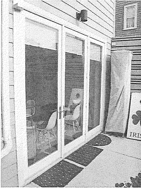
Figure 19: North side ground level.
