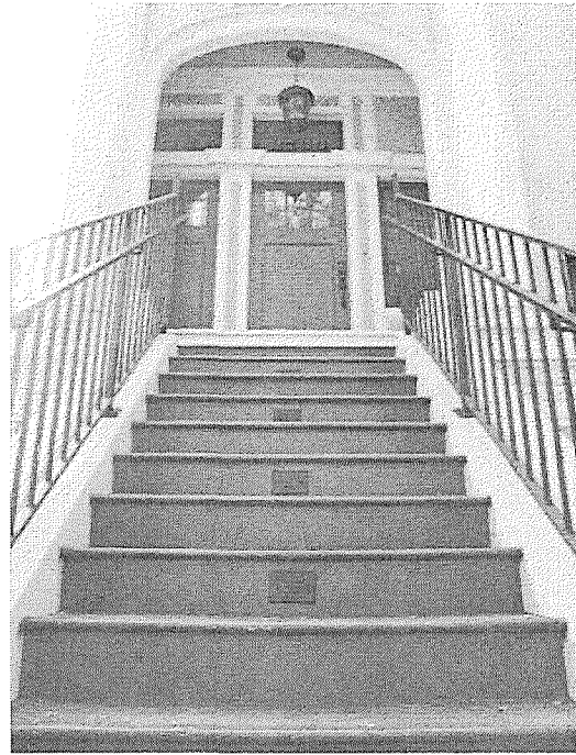
Figure 6: Exterior stairs leading to second story.
