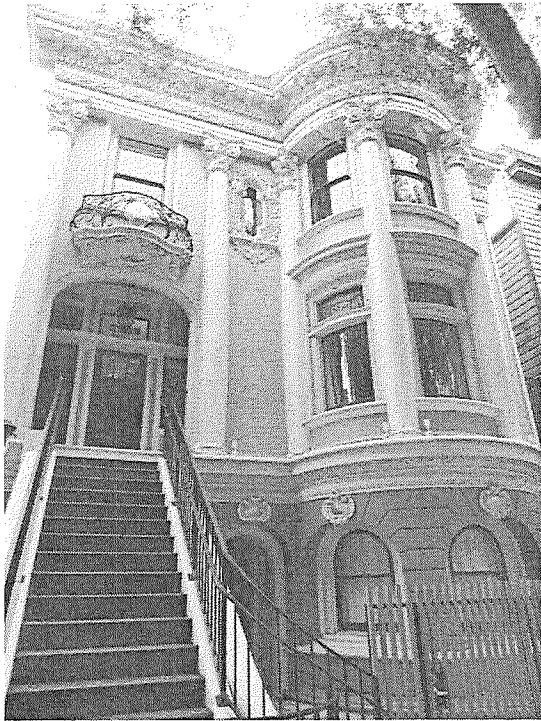
Photo 2: Front facade Looking east
