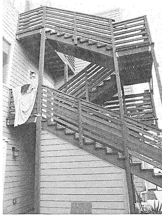
Figure 18: Exterior three-story stairs.
