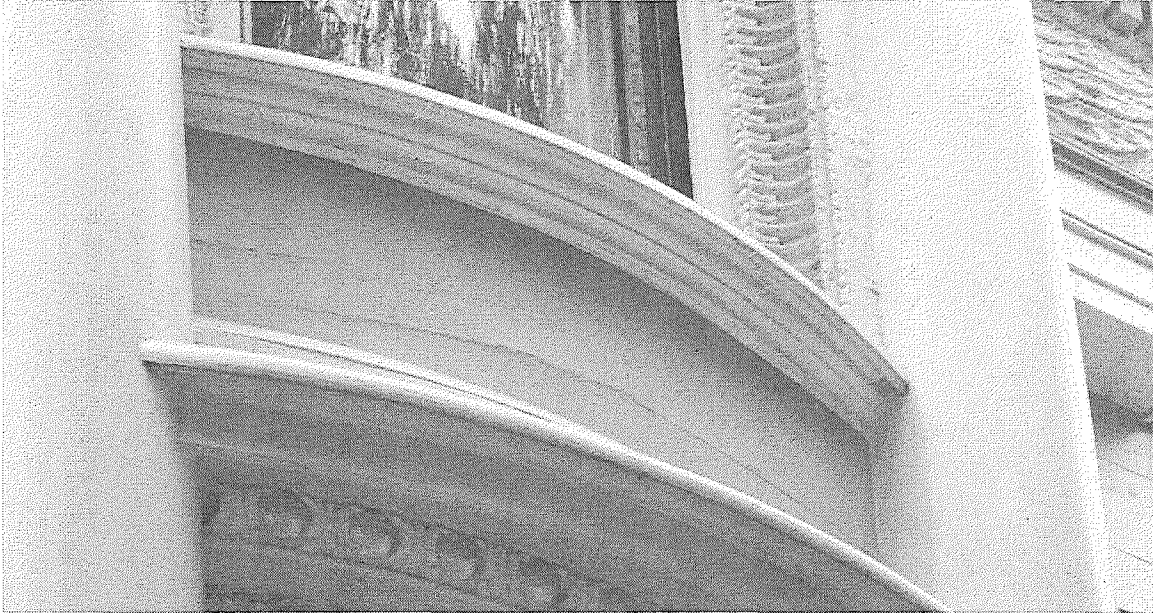
Figure 26: Detail of split wood panel between windows.
