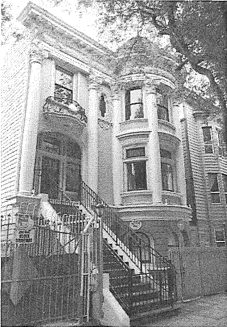
Figure 21: Primary (west) façade.
