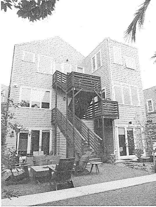
Photo 4: Rear facade Looking west
