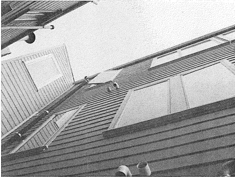
Figure 16: Second and third story fenestration of south façade.
