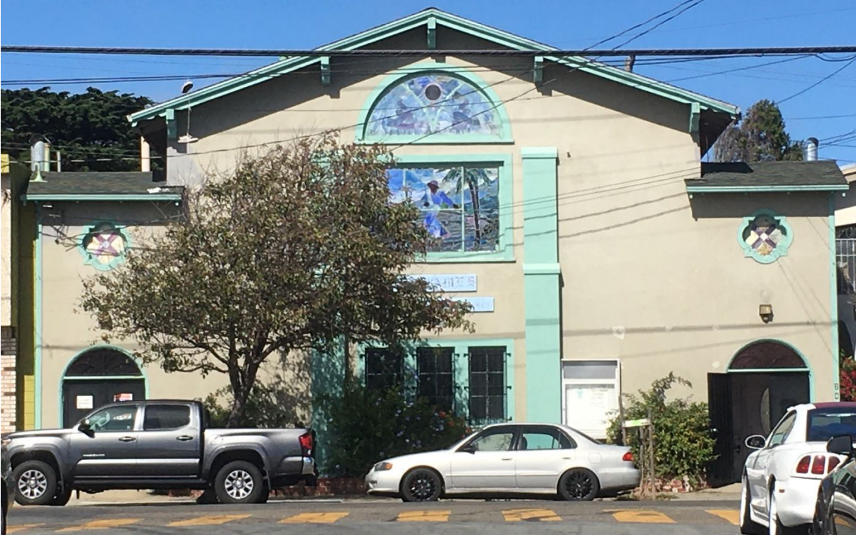
St. James Presbyterian Church, front (south) façade, view north, 2022 Source: San Francisco Planning Department
