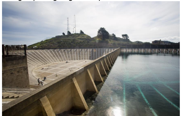
Twin Peaks Reservoir joint sealant
