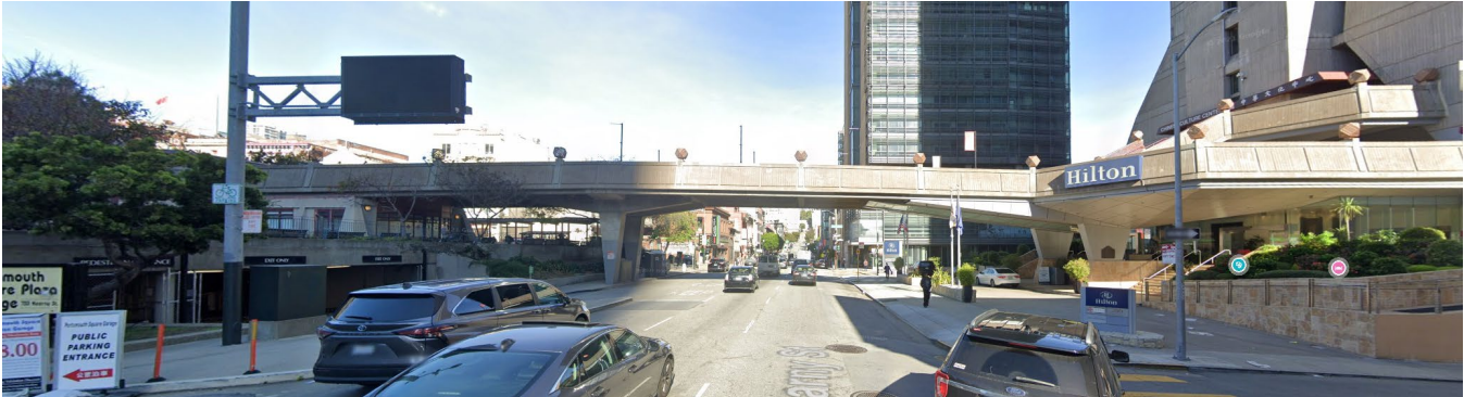
Figure 2: View of Pedestrian Bridge Looking North
