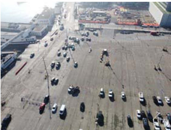
Aerial – Facing South
