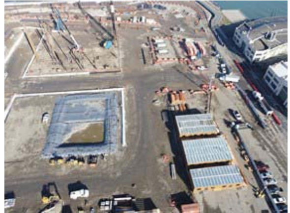
Aerial – Facing North
