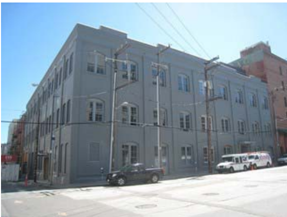
Lease 5 275 Brannan Street
