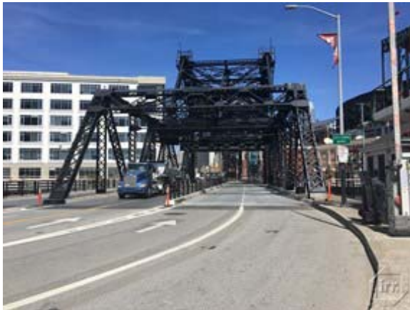
3rd Street – Facing North
