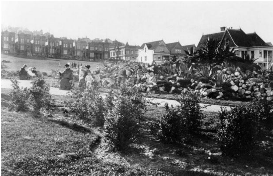
View from 1904 of the Duboce Park rock gardens. In the background are district houses on Carmelita Street.
