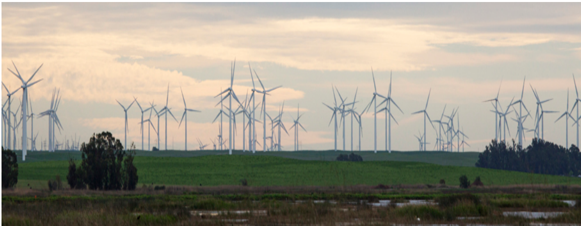
Photo 9: Shiloh I Wind Farm
