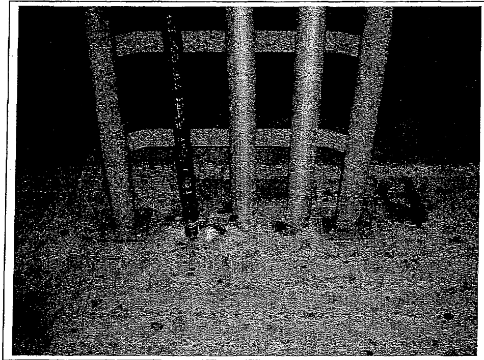
Proposed location of core drill from 2 nd level parking down into Sprint store. Note that there are existing core drills and a protective cage at this location.
