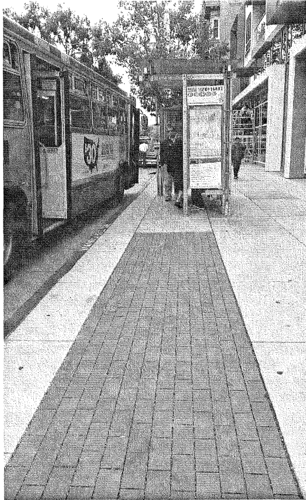
Permeable pavers along Van Ness Ave in San Francisco, CA. Photo: Krystal Zamora
