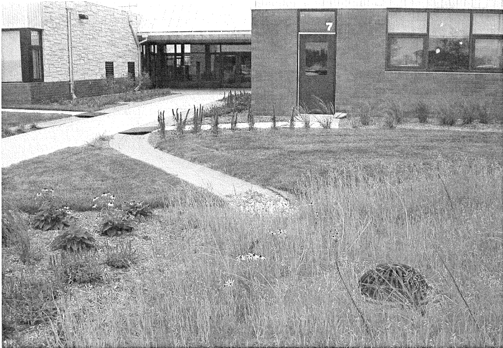
An impervious gutter directs roof runoff to a rain garden. Photo: Ken Kortkamp
