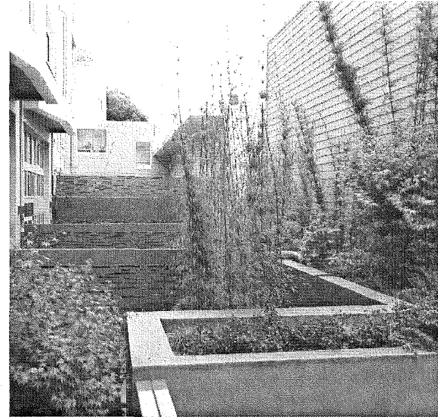
Bioretention planters are featured in private patios of a condominium development in San Francisco, CA. Photo: Krystal Zamora
