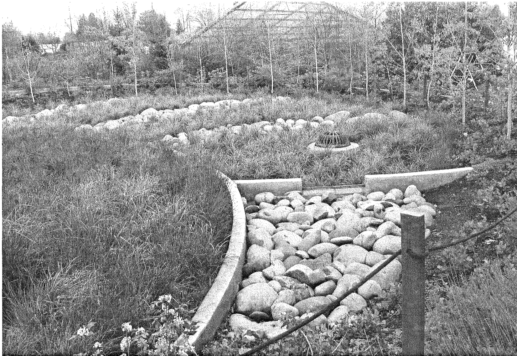
A rain garden at Glencoe Elementary in Portland, Oregon reduces stormwater flows to Portland's wastewater collection system. Photo: Rosey Jencks
