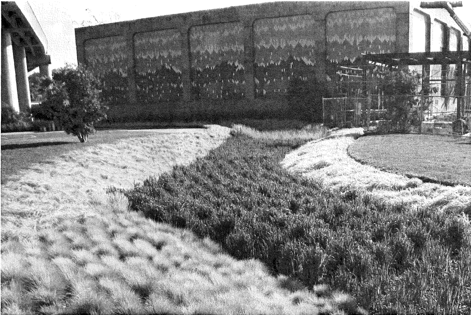
A swale in front of the San Francisco Public Utilities Commission's Channel Pump Station slows and treats stormwater before entering the Bay. Photo: Final citation pending
