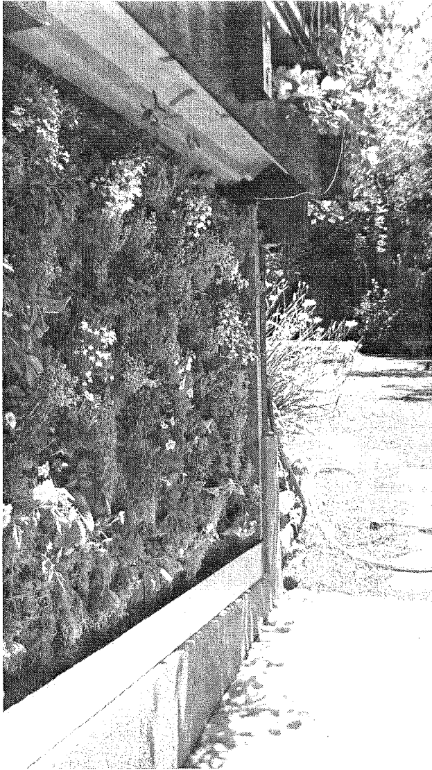
This green wall in San Francisco, CA is irrigated using captured stormwater. Photo: Rachel Kraai
