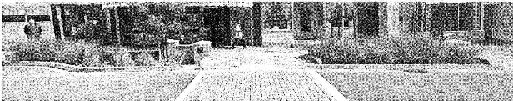
The Newcomb Ave Streetscape Improvement Project created one of the first streets to include green infrastructure in San Francisco, featuring bioretention and permeable pavement in an underprivileged neighborhood. Photo: Robin Scheswohl
