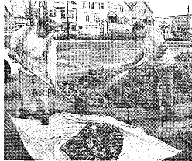
Maintenance workers remove sediment from a sediment basin in a bioretention planter on Cesar Chavez St in San Francisco. Photo: Robin Scheswohl
