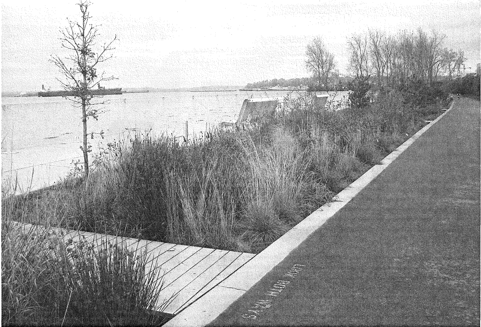
Boardwalks provide access across waterfront bioretention facilities in Seattle, WA. Photo: Rosey Jencks
