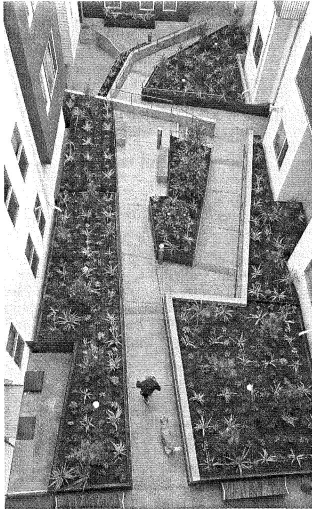
Bioretention planters in a residential courtyard in San Francisco, CA. Photo: Krystal Zamora
