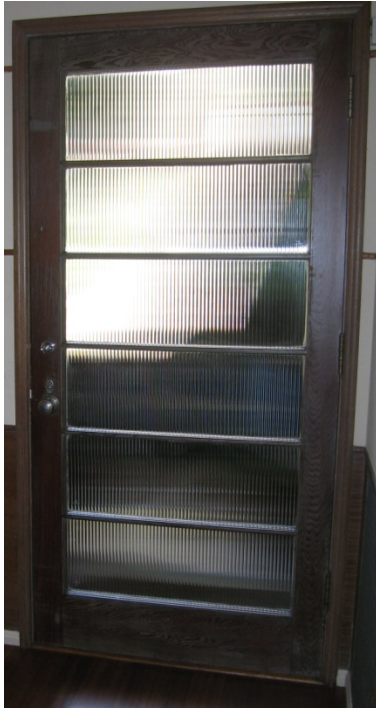
Left: Interior door with ribbed decorative glass set in horizontally oriented muntins (2012). Below: View of the living room looking north (2015).
