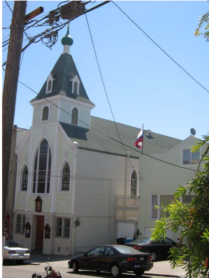
View from the northwest
