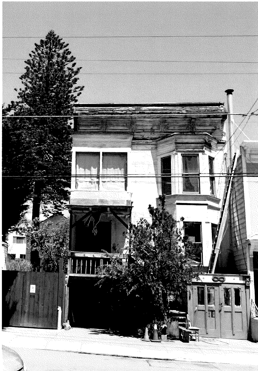
Current image showing subject tree located in different location than that shown in the circa 1946 image.
