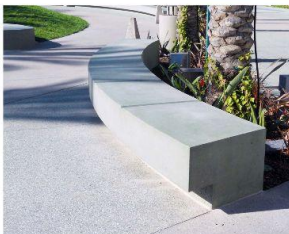
CONCRETE SEATWALL - FLAIN, SANDBLAST FINISH
