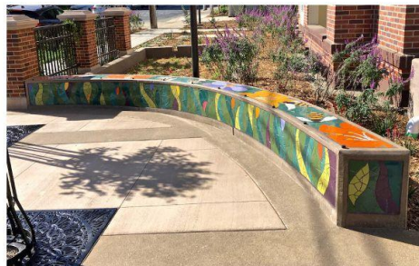
CONCRETE SEATWALL - WITH MOSAIC ARTWORK
