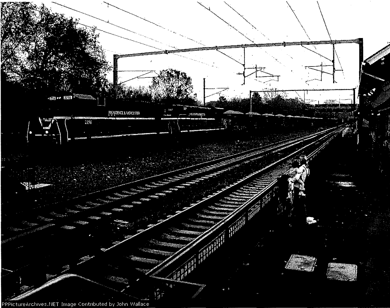
1 Figure B: Photograph of Providence and Worcester freight railroad operating on shared 2 tracks with electrified 25 kV overhead contact system overhead on the Northeast Corridor
