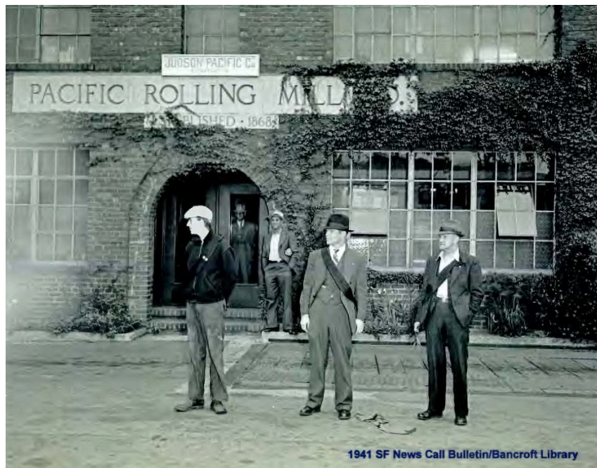
Figure 1: Three men stand alongside a grade-level truck scale in front of the Judson-Pacific Co. building at 1200 17 th Street. Extant building features include: the brick facade, sills, and arched portal; multi-light steel sash windows; and cast-cement sign. The sign notes the company's establishment date as 1868. Image dated 1941. Source: Bancroft Library, University of California, Berkeley.
