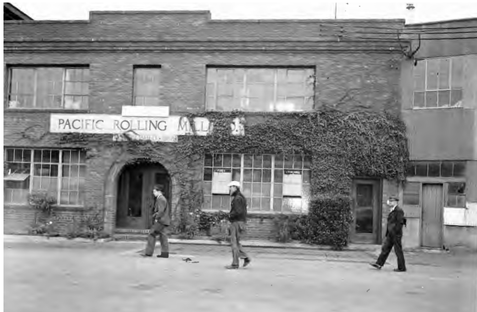
Figure 3: Brick and corrugated steel buildings at 1200 17 th Street. Note the corrugated steel façade of the warehouse at right. Image dated 1941. Source: Bancroft Library, University of California, Berkeley.
