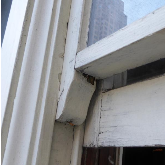
Figure 41: Detail photograph of window sash ogee lug (photograph taken on 02/27/2018).
