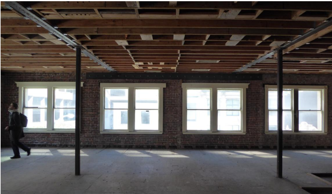
Figure 37: Photograph of typical east interior elevation (photograph taken on 02/27/2018).
