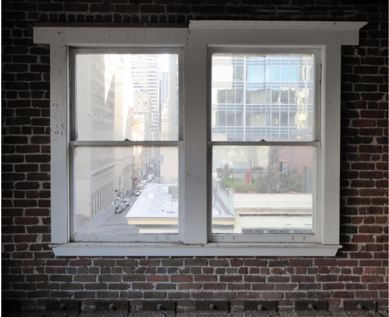
Figure 38: Detail photograph of typical double-hung windows at north and east walls (photograph taken on 02/27/2018).
