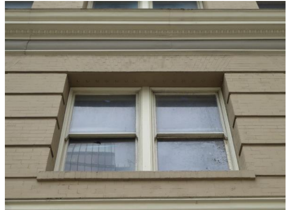
Figure 15: Photograph of typical punched window opening and painted brick cladding (photograph taken on 01/26/2018).
