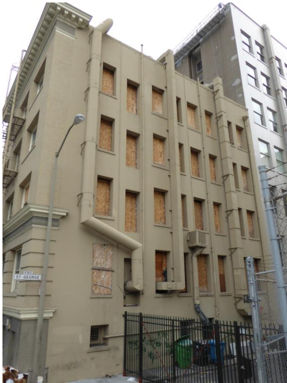
Figure 21: Photograph of St. George Alley elevation. Note punched window openings are boarded up with plywood at interior (photograph taken on 01/26/2018).
