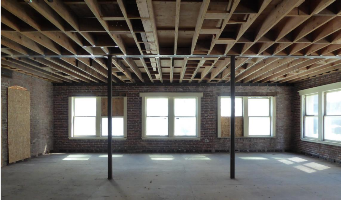
Figure 36: Photograph of typical north interior elevation (photograph taken on 02/27/2018).
