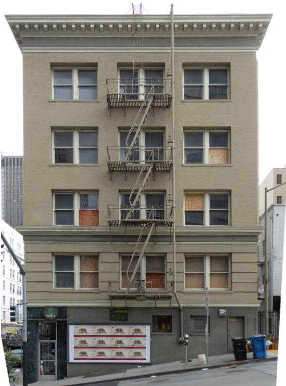
Figure 18: Photograph of Pine Street elevation with contemporary storefront at easternmost bay, and extant metal fire escape (photograph taken 01/26/2018).
