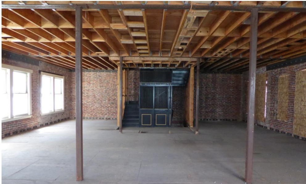
Figure 29: Photograph of typical south interior elevation. (photograph taken on 02/27/2018).
