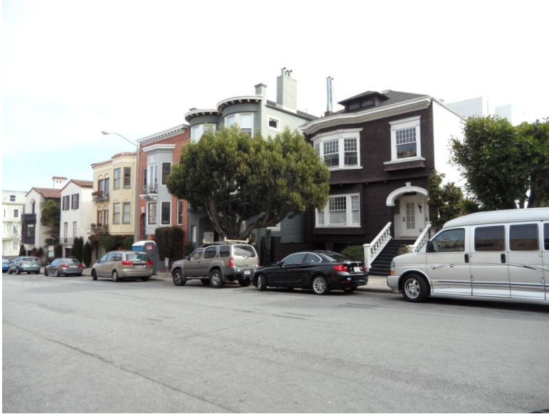
East side of Pierce Street looking north.
