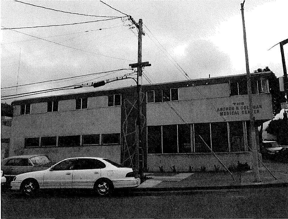
North (Ingerson Avenue) elevation, view south.
