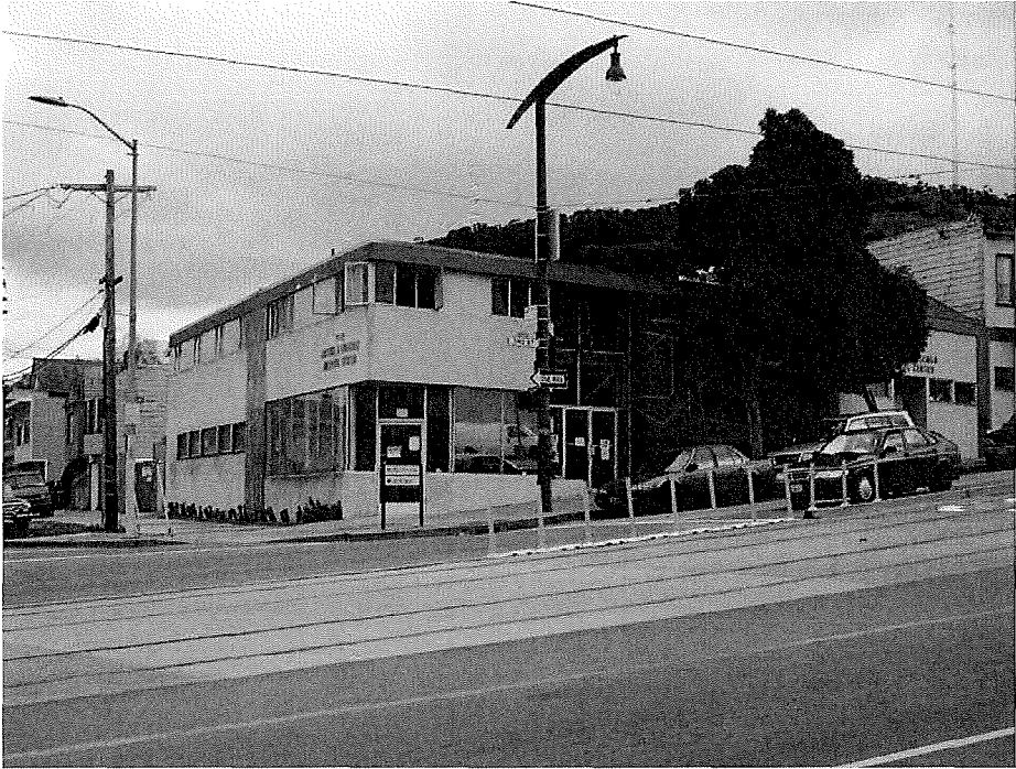
Primary (north and west) elevations, view southeast.
