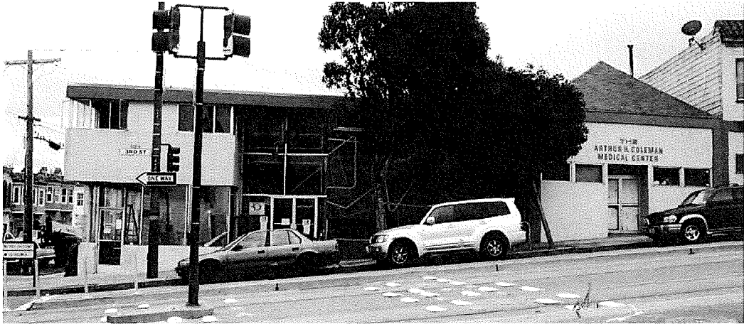
Primary (west) elevation, view east.
