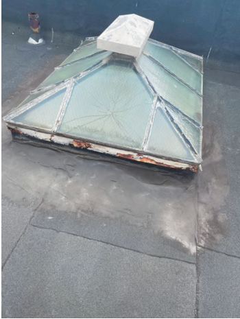
ROOF - SKYLIGHT ABOVE STAIR AT ELM STREET
