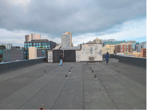
ROOF - VIEW TOWARD TURK STREET
