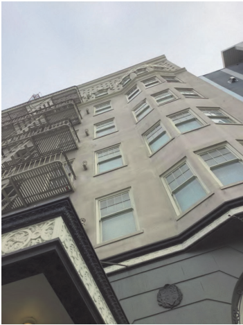
TYPICAL WINDOWS @ TURK STREET
