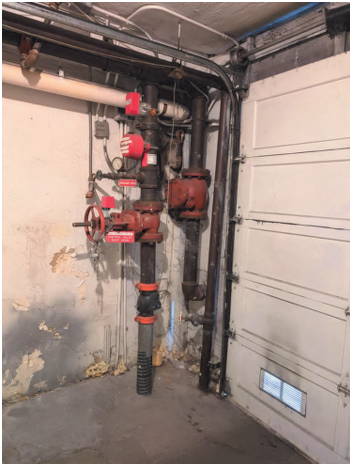
GROUND FLOOR - FIRE WATER ASSEMBLY
