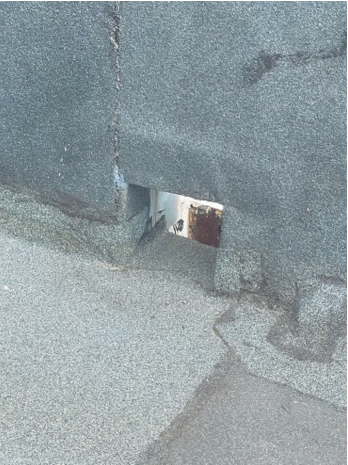
ROOF - EXISTING SCUPPER
