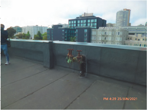
ROOF - FIRE WATER ASSEMBLY
