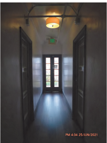
CORRIDOR - VIEW TOWARD TURK STREET
