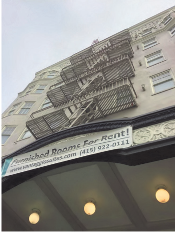
TURK STREET - FIRE ESCAPE
