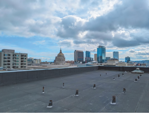
ROOF - VIEW TOWARD ELM STREET
