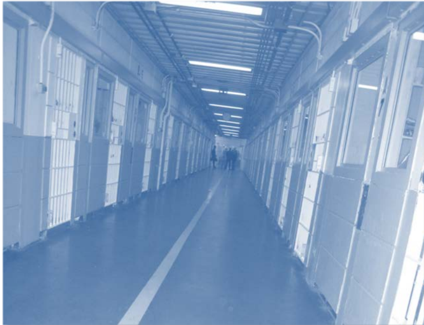
Unsafe County Jail #4
