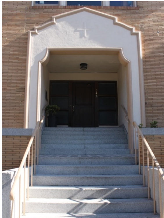
FIGURE 39 (LEFT). RECTORY: MAIN ENTRANCE, 2015.
