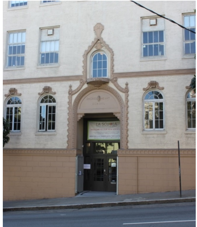
FIGURE 44. SCHOOL: MAIN ENTRANCE, 2015.
