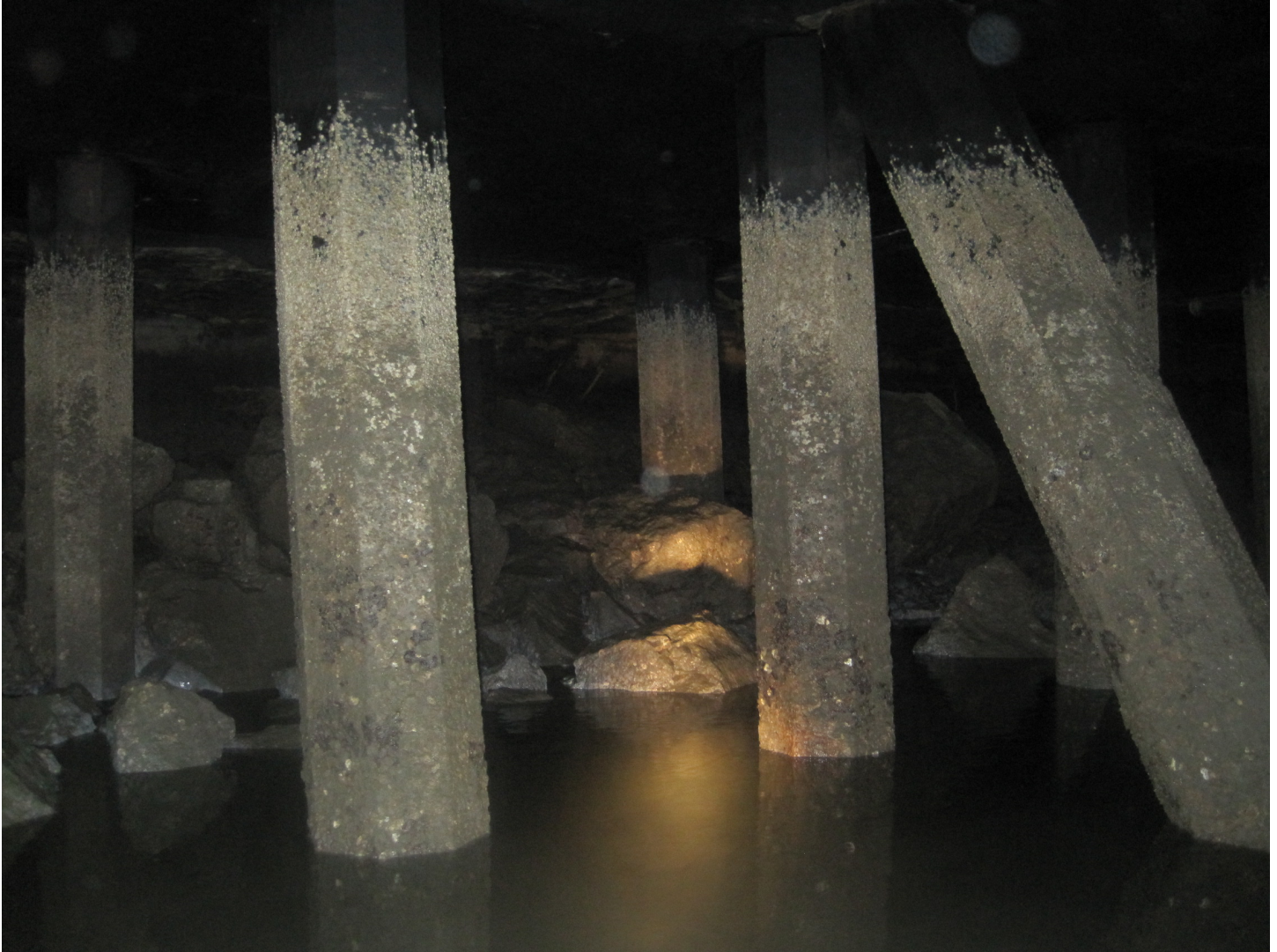
Photo 7. Seawall protected by rip-rap
