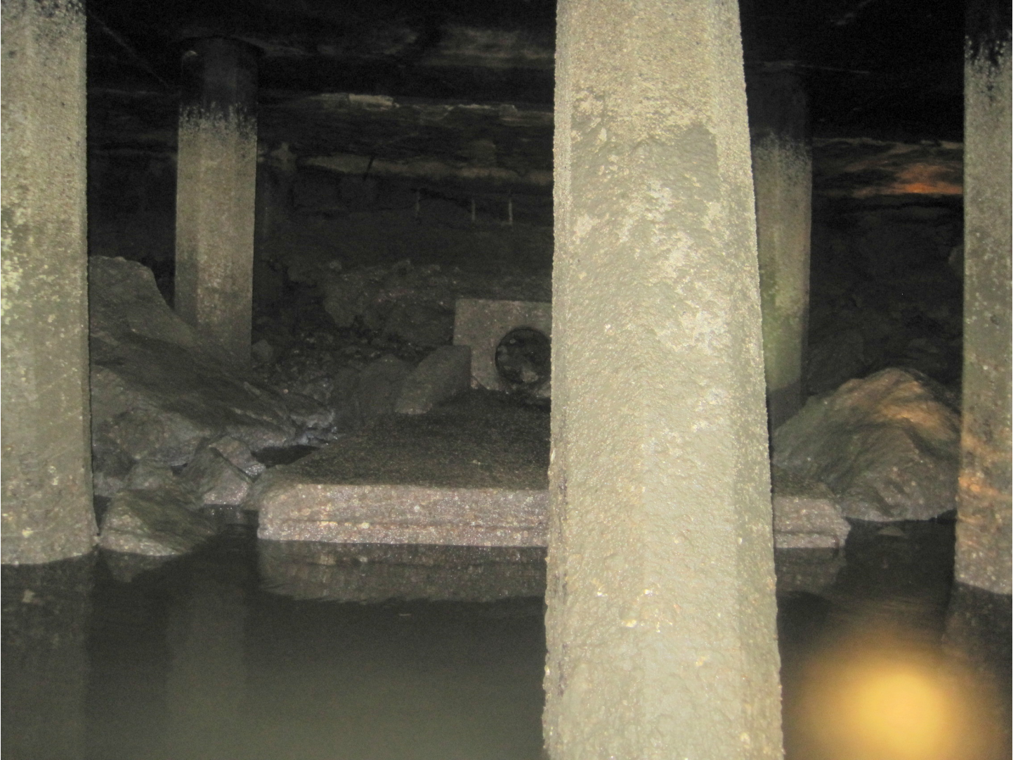
Photo 2. Drain underneath seawall
