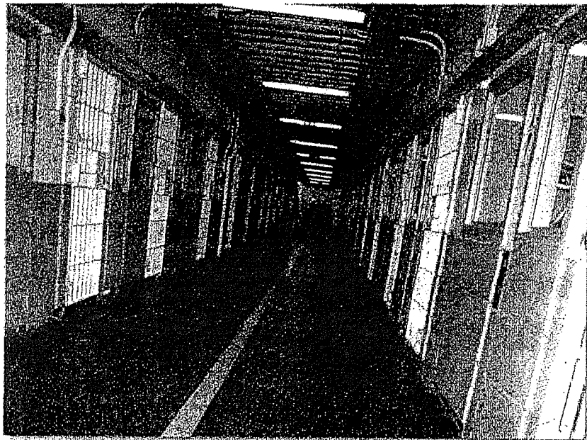
Unsafe County Jail #4
