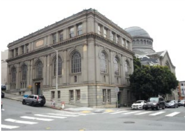
North and West elevations (HRE)
