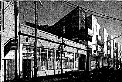
Diversity of Buildings and Architecture
