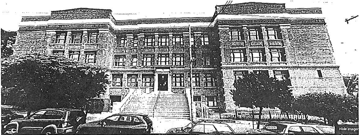
Figure 87. Former Lowell High School (now San Francisco City College's John Adams Campus).
