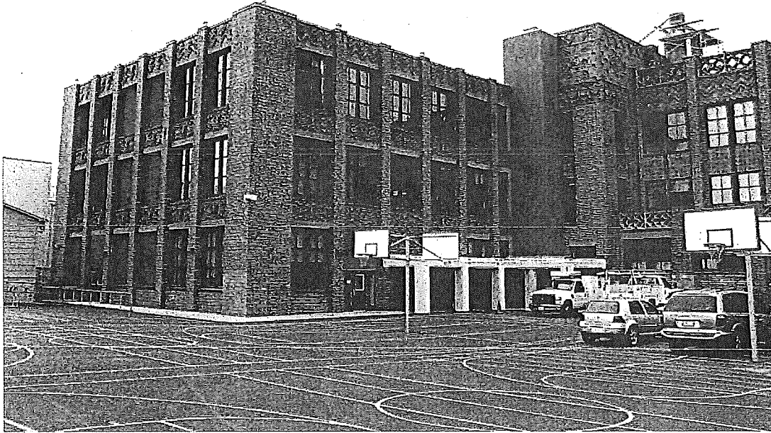
Figure 28. East façade (south section) of Theodore Roosevelt Middle School; view toward southwest.
