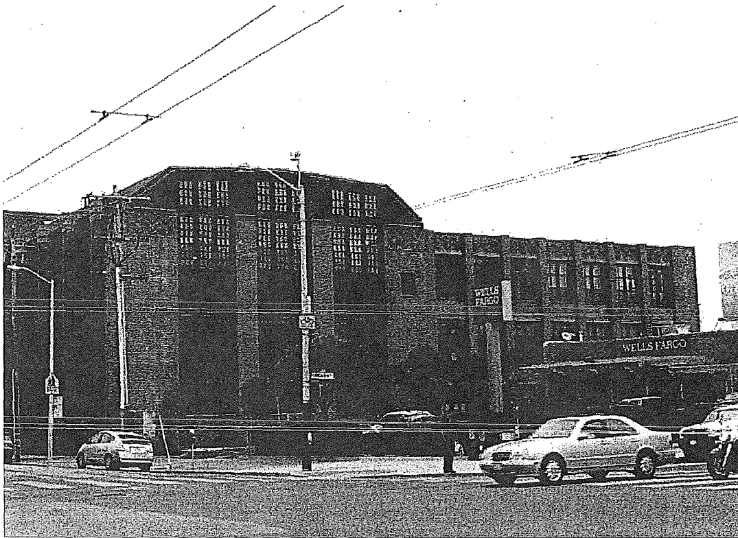
Figure 27. South façade of Theodore Roosevelt Middle School; view toward northeast.
