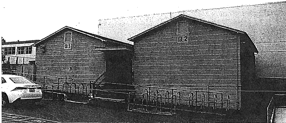
Figure 57. Temporary classrooms at southeast corner of campus; view toward southeast.
