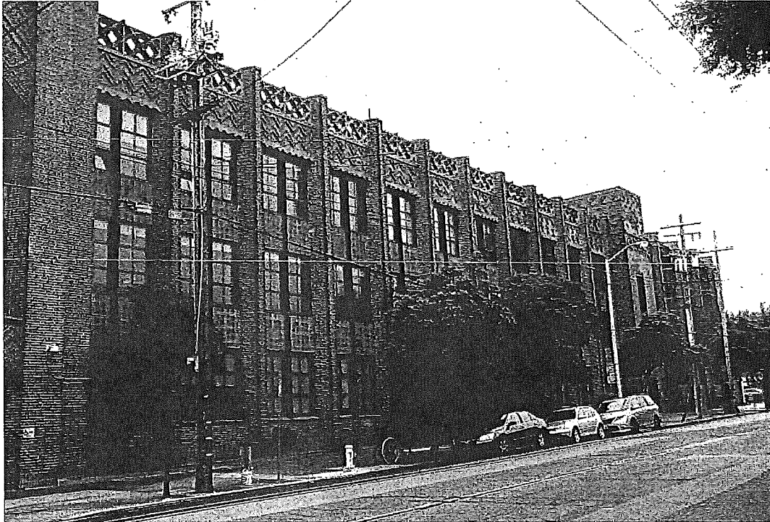
Figure 23. Academic building; view toward southeast.
