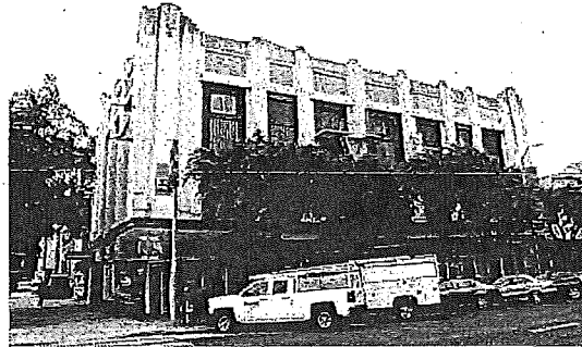
Figure 3. 1 Clement Street, built 1908 and remodeled ca. 1930; view toward south.
