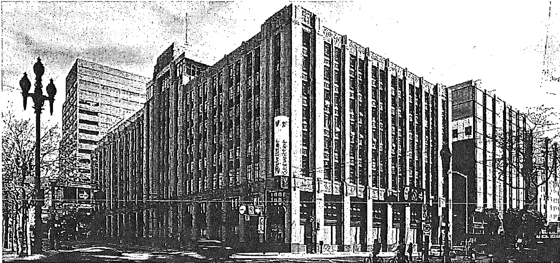
Figure 79. Western Furniture Mart, by The Capitol Co., Architects, 1937.
