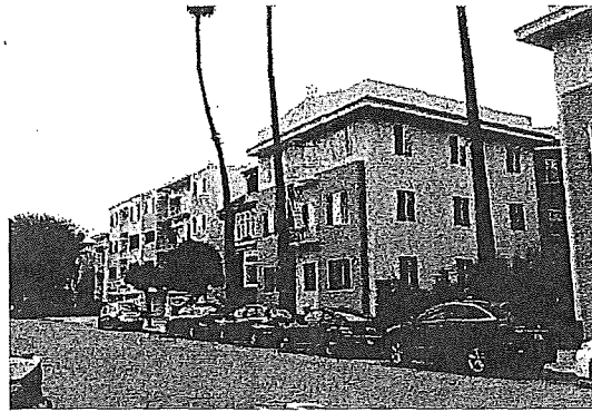
Figure 11. West side of Palm Avenue north of Roosevelt School; view toward south.
