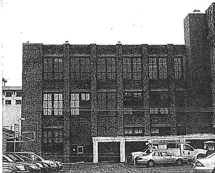
Figure 33. North façade of gymnasium wing of Theodore Roosevelt Middle School; view toward south.
