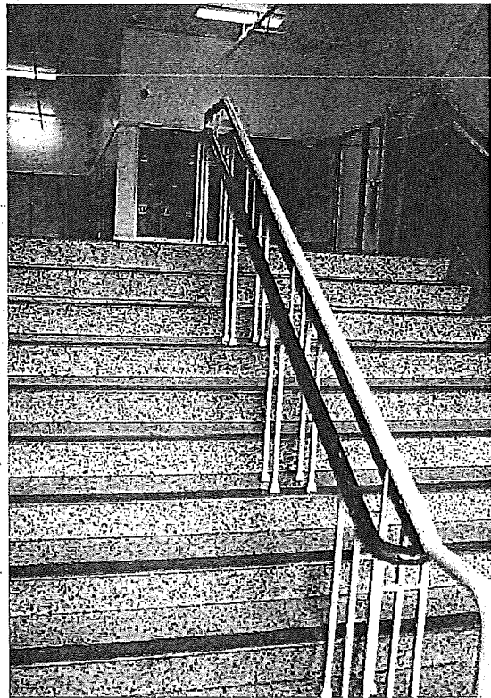
Figure 43. North stair between first and second floor levels.
