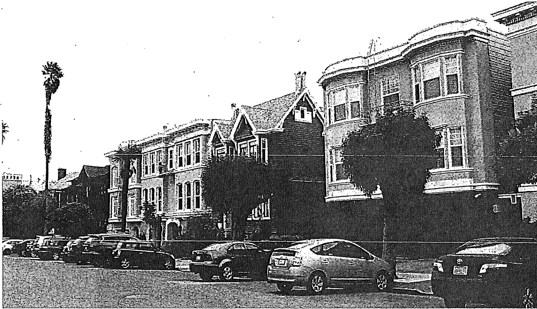
Figure 13. East side of the 100 block of Palm Avenue; view toward northeast.
