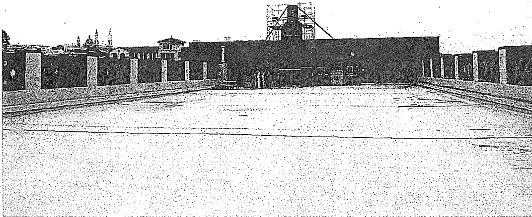
Figure 54. Rooftop play area; view toward north.
