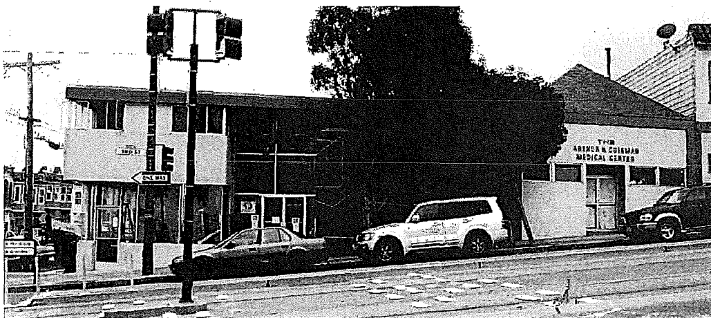
Primary (west) elevation, view east.
