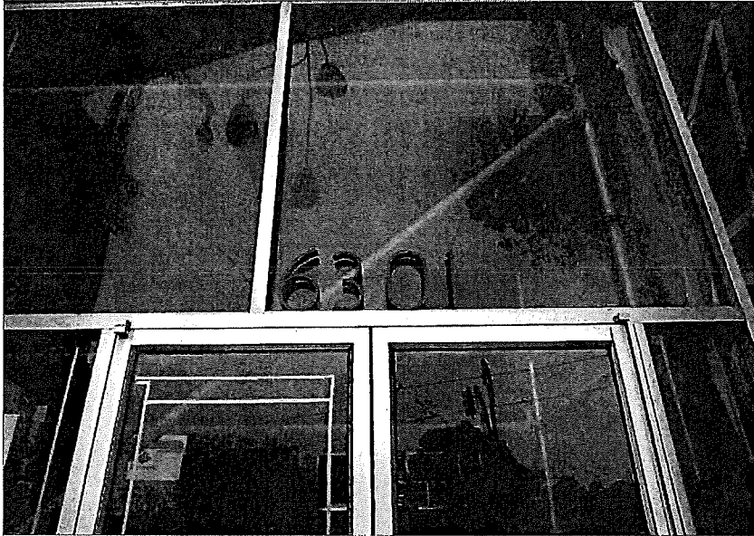
Detail of metal numbers above Third Street entrance, view east.
