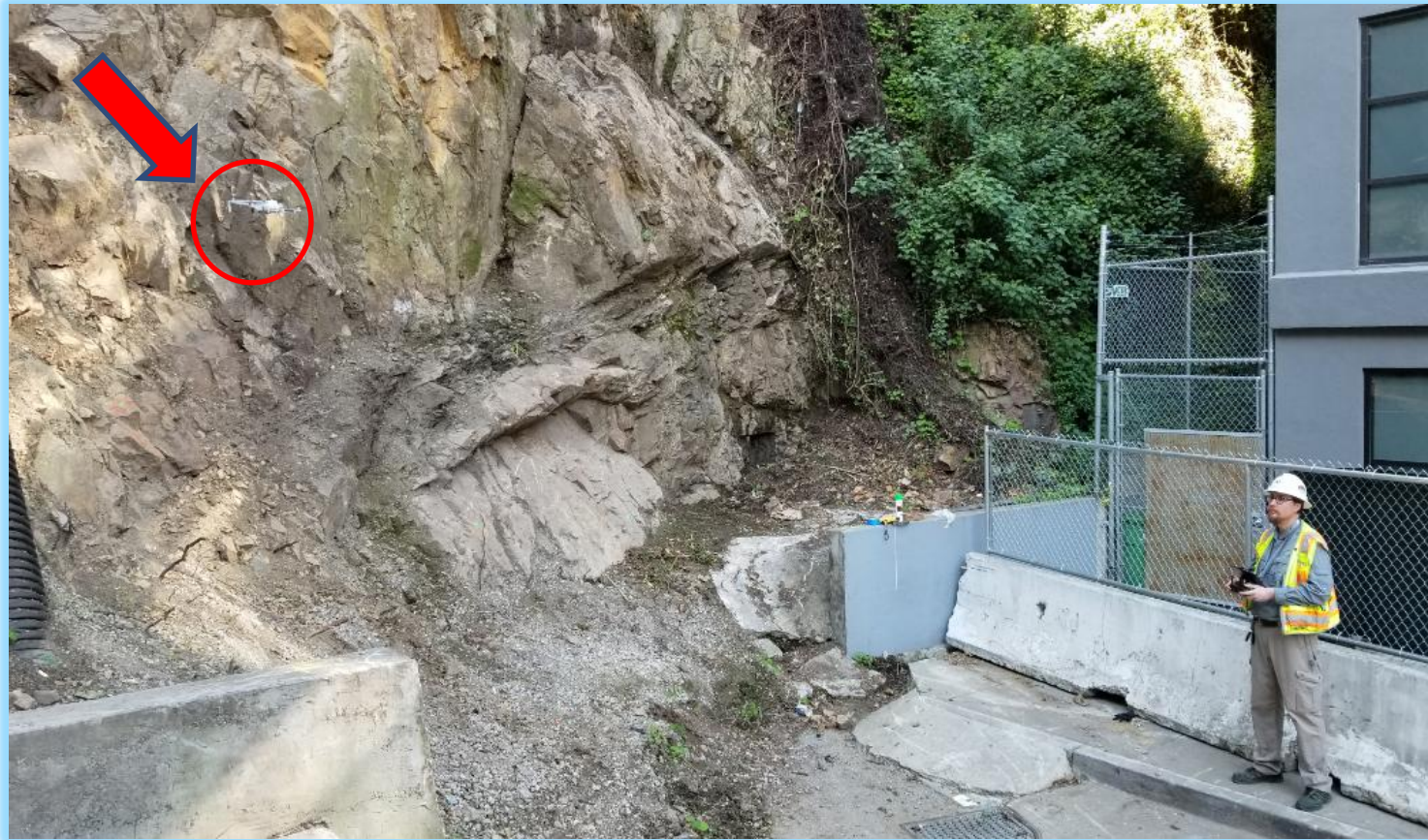
Photo: Filbert Street hillside inspection, 2019
