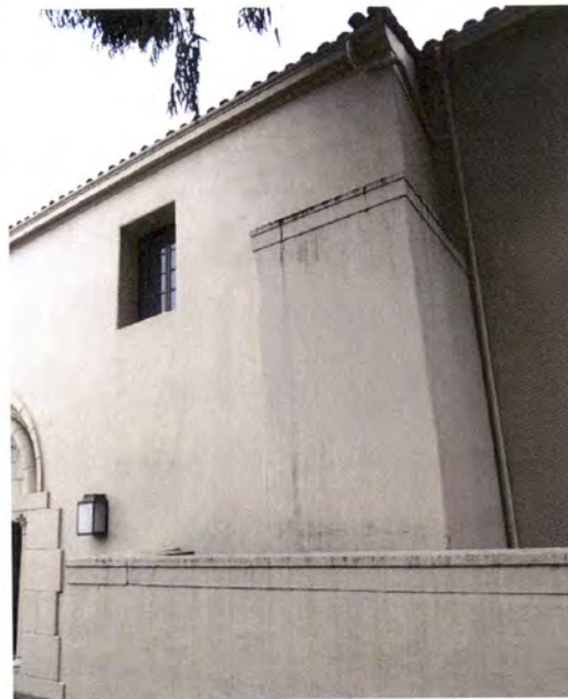
Figure 23 - Areas under this tree on Haight Street could be cleaned, and will require it more regularly than others on the facade. Photo by Page & Turnbull
