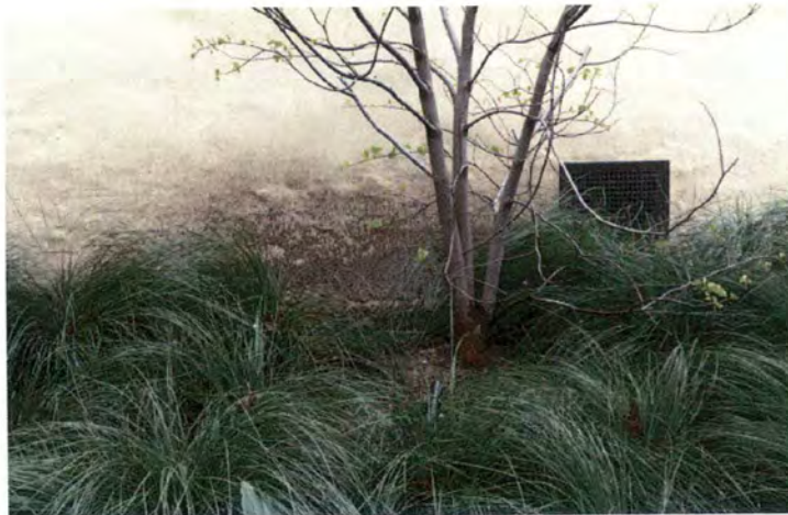
Figure 14 - Splashback on the exterior walls. Photo by Page & Turnbull, 2017.
