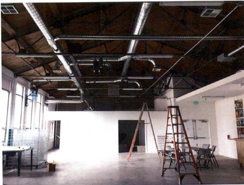
Figure 28 - Second floor workspace with exposed trusses and sheathing
