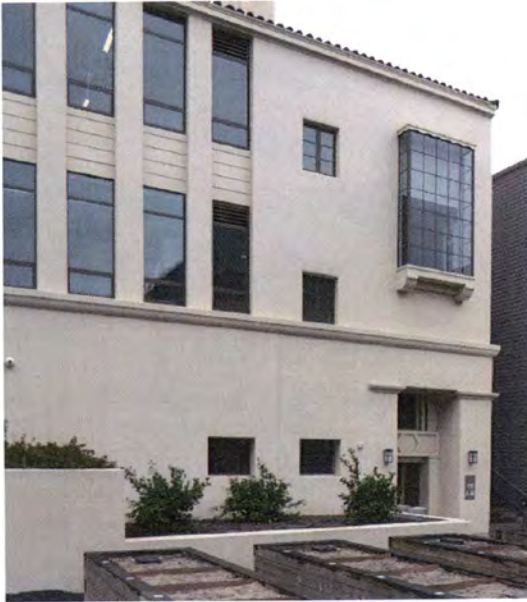
Figure 20 - Variety of windows on the south facade, all in good condition after the rehabilitation. Photo by Page & Turnbull
