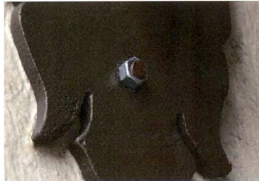
Figure 15 - (above) A rusting bolt anchoring the sconces. Photo by Page & Turnbull, 2017
