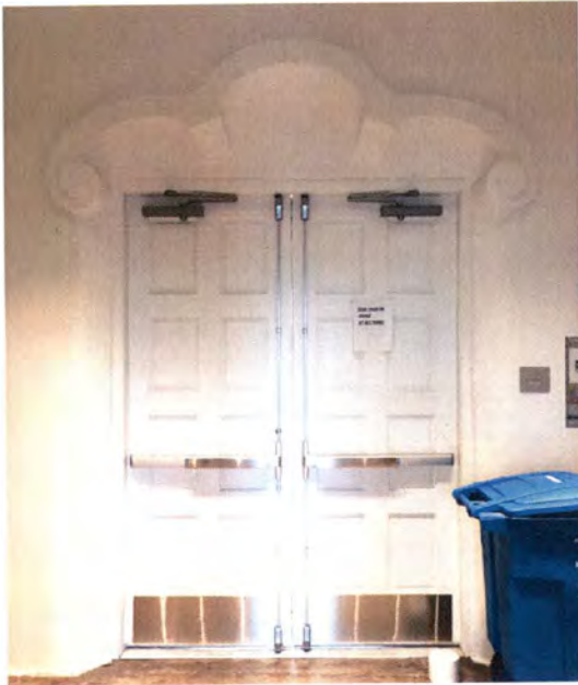
Figure 26 - Haight Street entry interior
