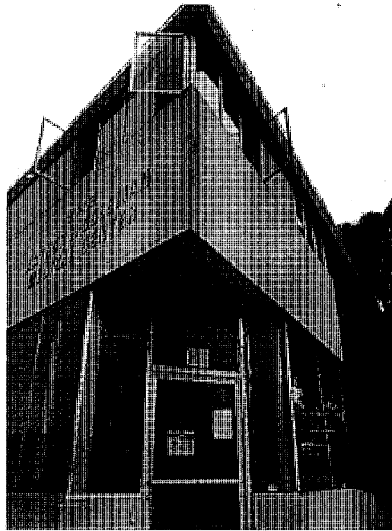
North entrance at corner of Ingerson Avenue and Third Street, view southeast.
