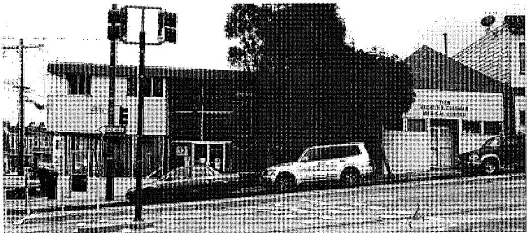
Primary (west) elevation, view east.
