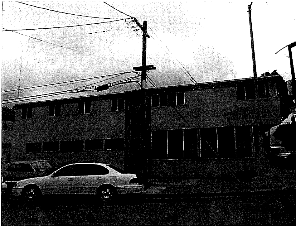
North (Ingerson Avenue) elevation, view south.
