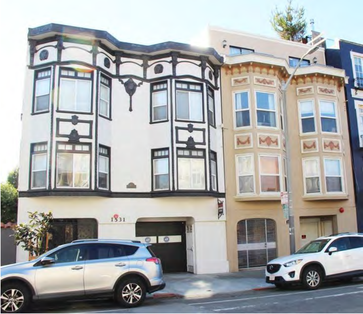
Figure 7. From left to right: 1531 (built 1924) and 1535 (built 1925) Francisco Street.
