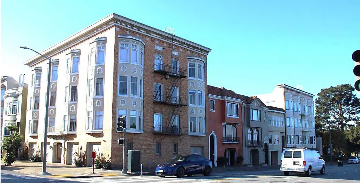
Figure 2. South side of Bay Street, including, from left to right: 3355 Octavia Street and 1415, 1421, 1425-27, and 1435 Bay Street – all built between 1924 and 1931.
