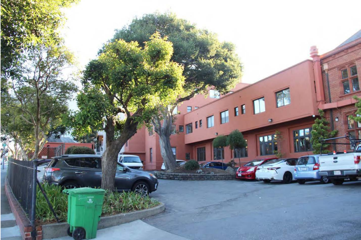
Figure 14. Parking lot at north side of property.
