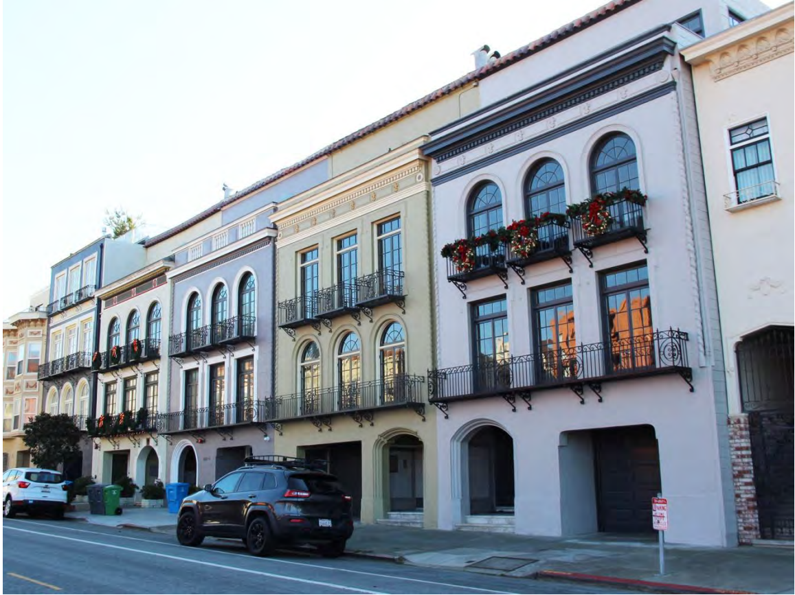
Figure 8. From left to right: 1547-49, 1553-55, 1557-59, 1561-63, 1567-69, and 1573-75 Francisco Street (all built between 1925 and 1927).
