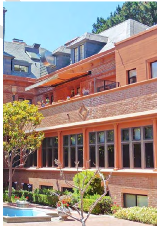
Figure 26. Juncture of (north) rear wing of Morgan Building and 1957 Perry Building. Source: Page & Turnbull
