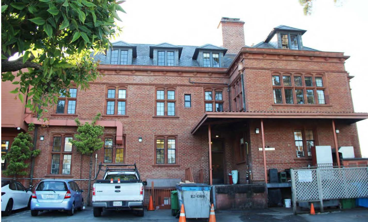
Figure 21. North (secondary) façade of the Morgan Building.
