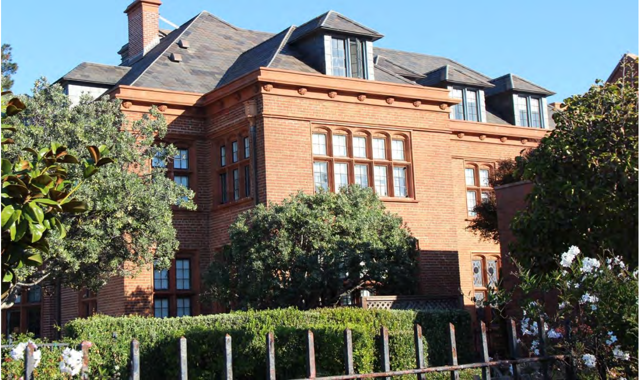
Figure 22. South (tertiary) façade of the Morgan Building.
