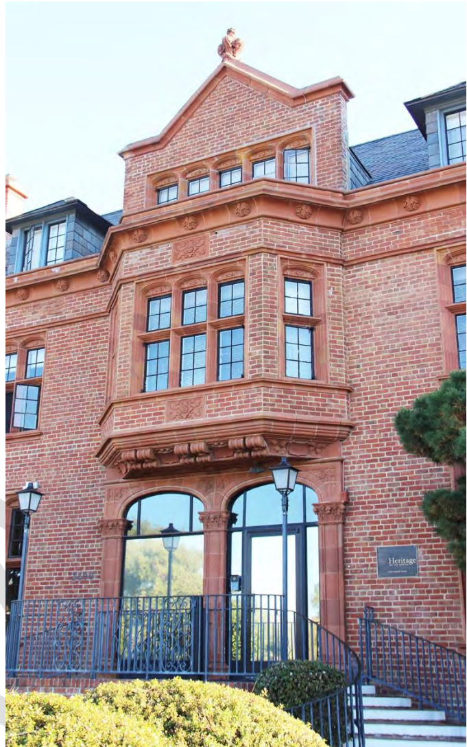
Figure 19. Main entrance with oriel above.
