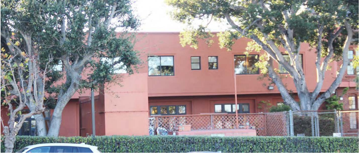
Figure 31. Linking wing of the Perry Building; view from Bay Street.
