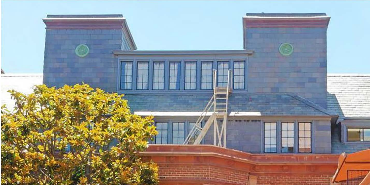
Figure 25. Penthouse and dormer on east façade. Source: Page & Turnbull
