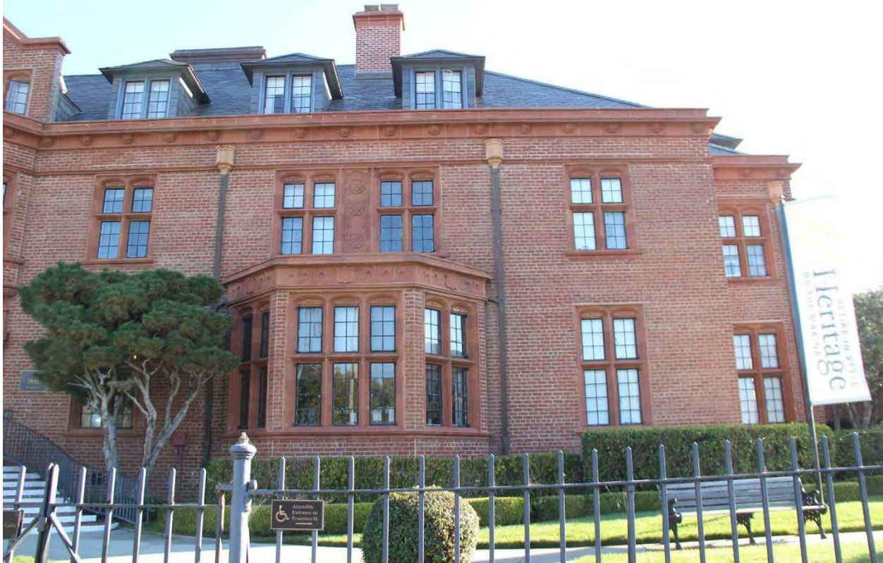
Figure 20. Detail of the primary façade – right (south) side.
