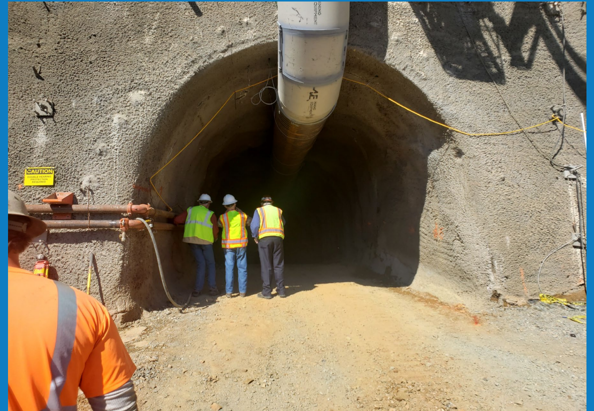
New Priest Adit Tunnel Under Construction
