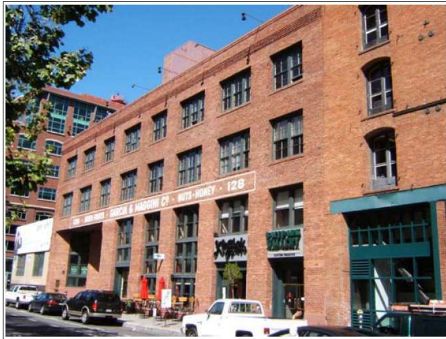
Garcia and Maggini Warehouse, 128 King Street
