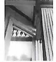
FIG. 2: EXISTING PORCH ROOF DRAIN PIPE
